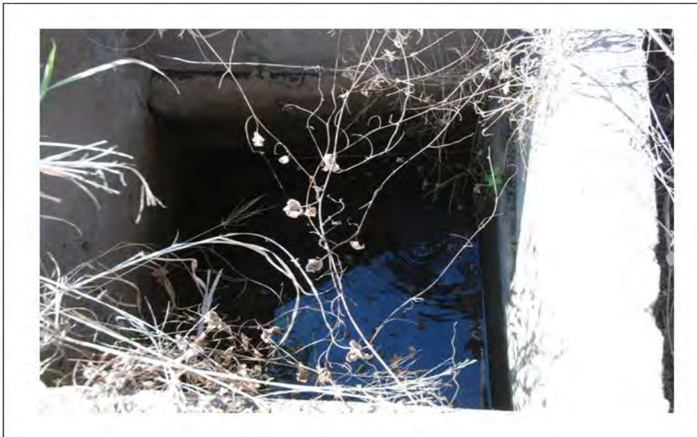
Figure 2.7 One of the uncovered and blocked man-holes at a sugarcane field with a poorly-maintained subsurface drainage system (PMDS)
