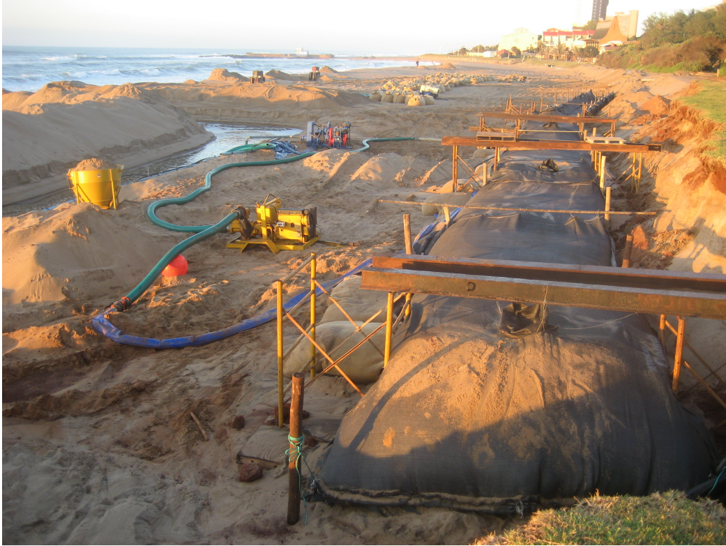
Figure 9.11: Geotextile tube installation at Amanzimtoti (April 2008)
