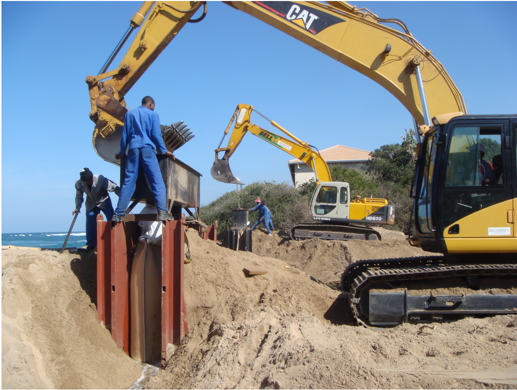
Figure 9.7: Filling of Geotextile Sand Bags with frame (April 2007)
