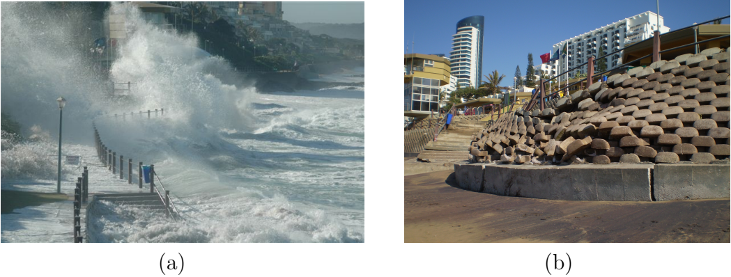
Figure 10.2: (a) Waves breaking on a loffelstein seawall in Umhlanga (03/07/2011) and (b) the subsequent failure of the loffelstein seawall (02/08/2011)
