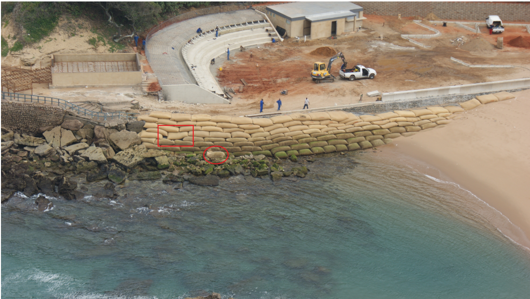
Figure 10.5: A geotextile bag seawall failure at Isipingo (July 2011). The red rectangle highlights where a bag was removed from the seawall and the red circle identifies the removed bag
