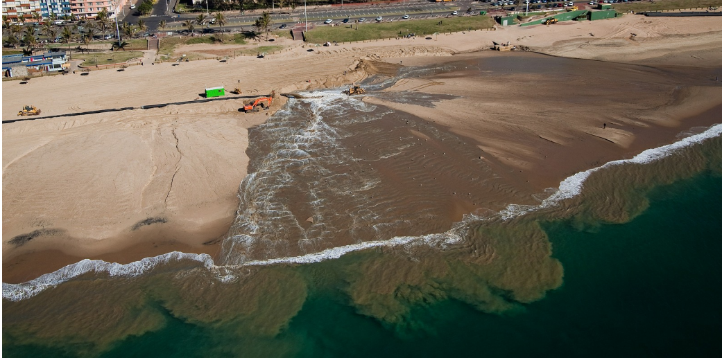
Figure 9.3: Beach nourishment at Addington Beach (Dredging International, June 2009)
