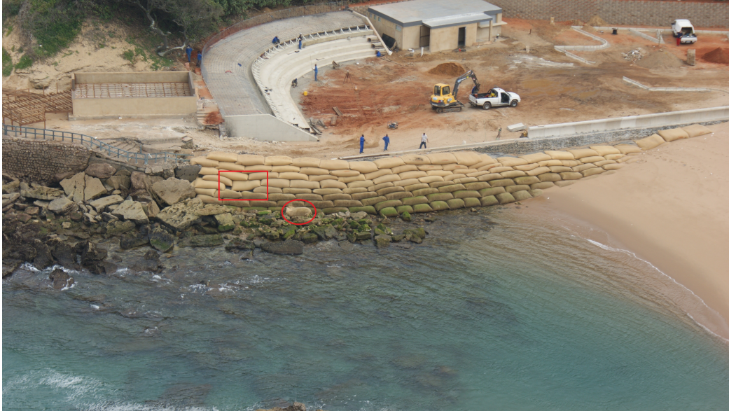
Figure 9.10: A geotextile bag wall failure at Isipingo (July 2011). The red rectangle highlights where a bag was removed from the wall and the red circle identifies the removed bag.
