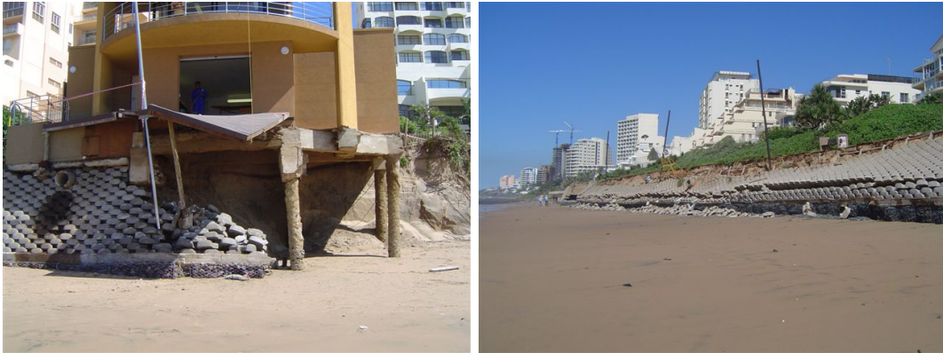
Figure 9.5: Failure of loffelstein seawall at Umhlanga main beach (eThekweni Municipality data base, 20 March 2007)
