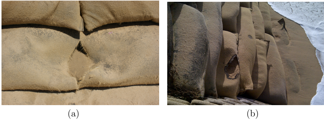
Figure 10.7: Geotextile sand bags that have been (a) cut and (b) burnt
