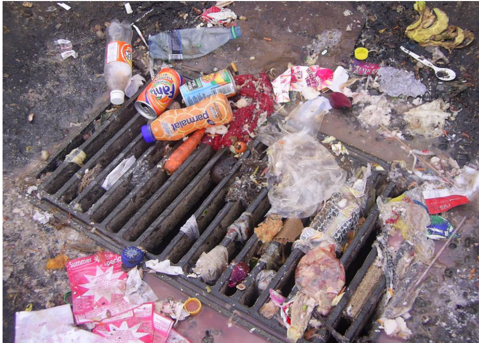
Picture 7-4: A storm water drainage system used to dispose of dirty water at the Limpopo Mall parking area
