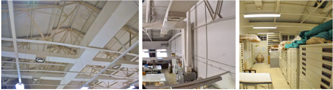
Fig.ii. 5 : Roof structure inside the beehall. Fig.ii. 6 : Stud dividing wall in the beerhall. Fig.ii. 7 : Inside the storage facility.
