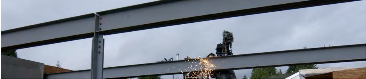
Fig_ii. 10 : Steel cruciform columns being used on a residential project.
