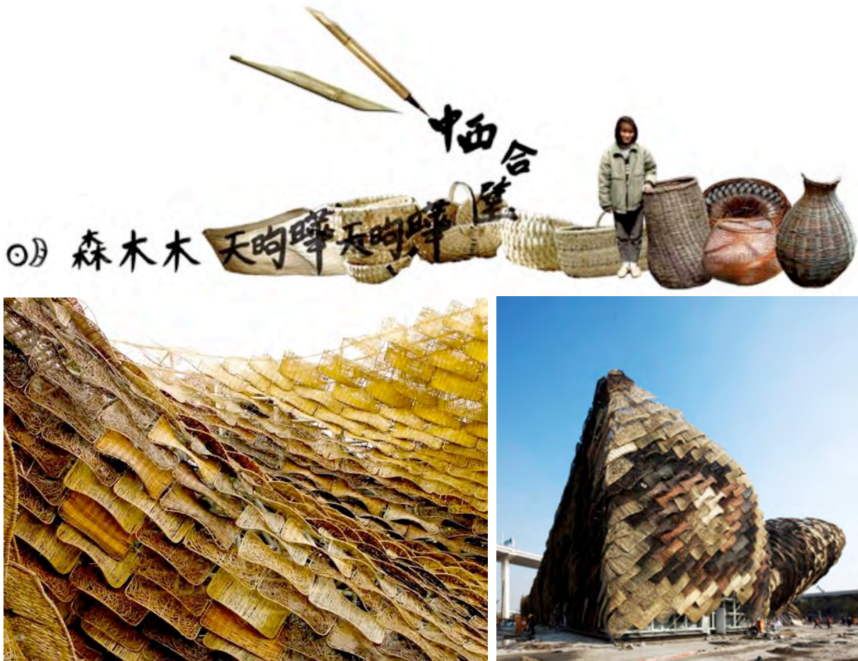
Fig_2.3. 5 : The formulation for the conceptual abstraction of basketry into a design for a handcrafted-architectural tectonic. Fig_2.3. 6 & Fig_2.3. 7 : Each panel is hand made and different to the next. Mass production through hand-made craftsmanship. Spanish Pavilion for Expo Shanghai 2010, Enric Miralles Benedetta Tagliabue.
