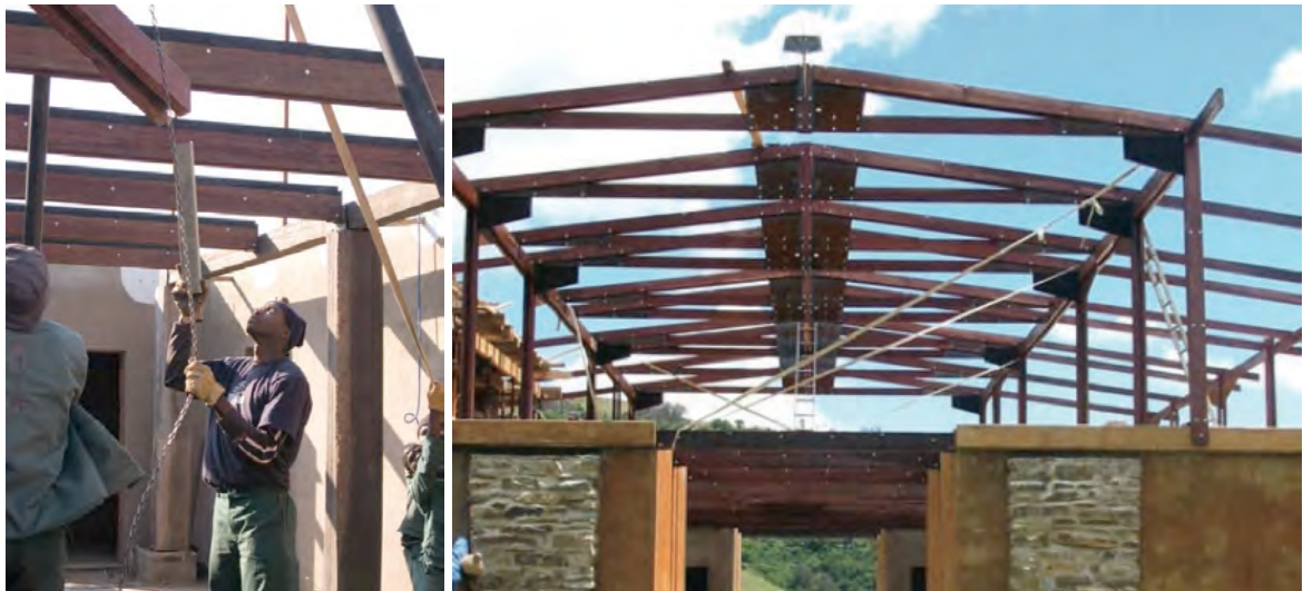
Fig_3. 22 : The architects were able to achieve longer spans by using steel gusset plates to brace the structures, which were essentially put together like a mecano set. This is one of Koop Architects principles of Design; treat architectural construction like big pieces of furniture. ( www.koopdesign.co.za ).
