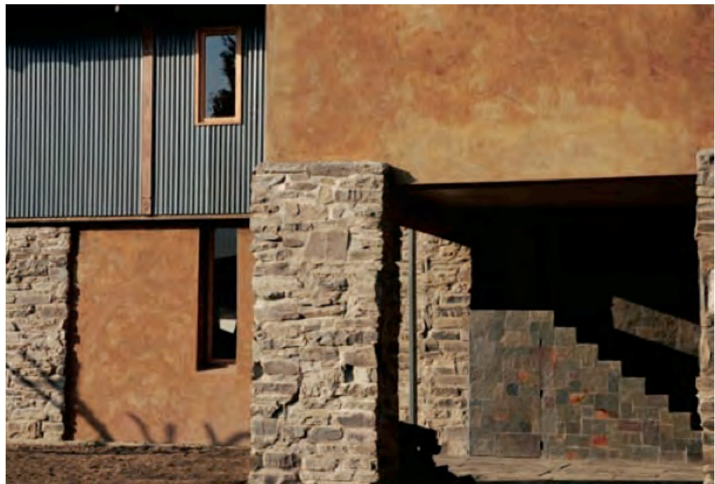
Fig_3. 26 : The material palette used for the Barn. Existing stone marks the previous buildings footprint. Colour bonded steel sheets are used as infill sections. Raw plastered brickwork blends into the colours found in the landscape. Bespoke joinery designed by Koop and built on site
