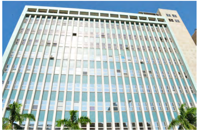
Fig_2.1. 13 : Air-conditioning ducts accessorize a building in the hot and humid environment on the east coast of South Africa, Durban.
