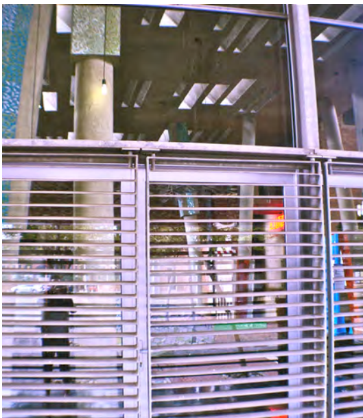
Fig_3. 4 : The screened ground floor allowing glimpses into the foyer
