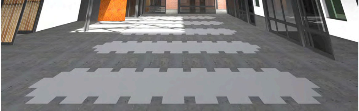
Fig_ii. 29 : Detail of the flooring in the beerhall, with vinyl inlays.
