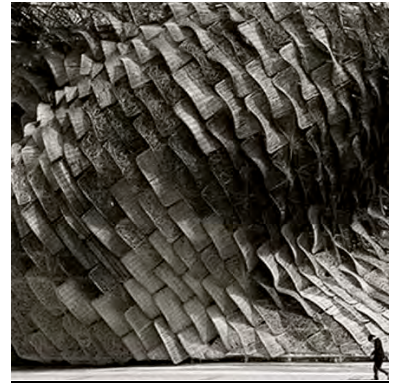
Fig_4.4 : Handcrafted mass production. Spanish Pavilion cladding. China.
