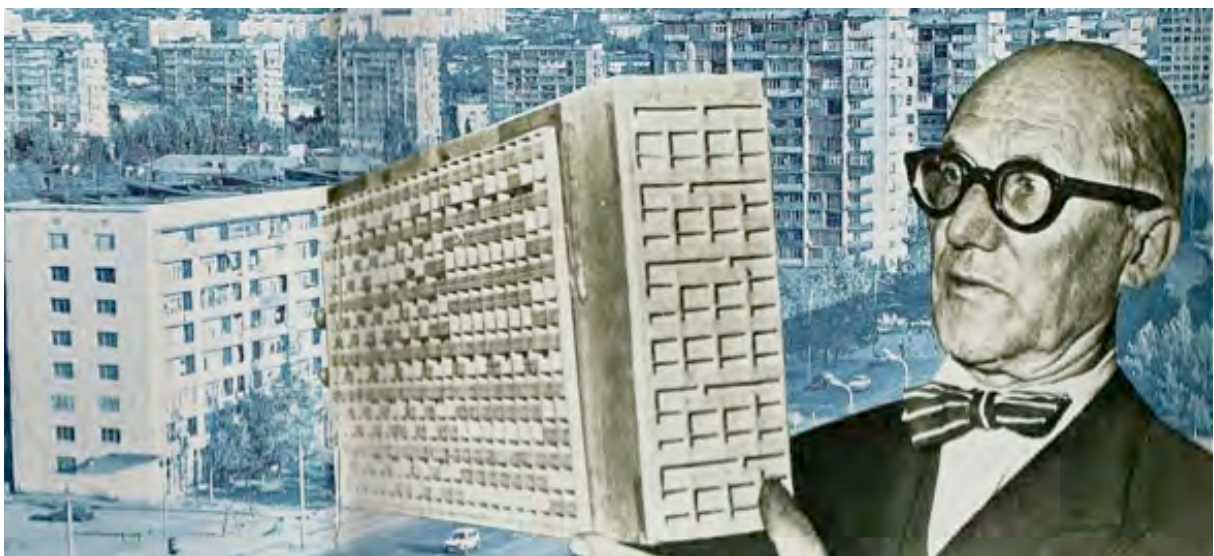
Fig_2.1. 3 : Montage of Le Corbusier holding a model of Unite D’Habitat. A mass produced Architecture formulated through Prefabricated units that would then “slot” into a concrete framework.
