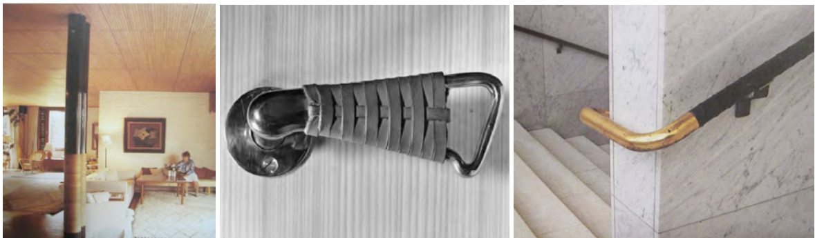
Examples of Aalto’s considerate design elements that aimed towards a balanced human encounter with typically machine made components. Fig_2.3. 11 : The custom door handles designed from Mason Louis Carre’ in 1959 encompass a leather bound grip. Fig_2.3. 12 : The detail of the Handrail at the Finladia Hal explores a machine made handrail wrapped leather in the areas where it will be in contact with a human hand. Fig_2.3. 13 : The columns Villa Maireia are wrapped with Rattan and are warm to the touch and create a sense of human consideration.
