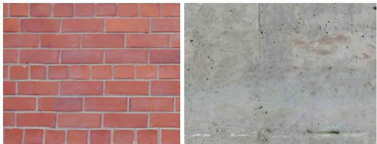
Fig_ii. 14 : Existing brickwork of the beer hall. Fig_ii. 15 : Existing concrete of the beer hall.
