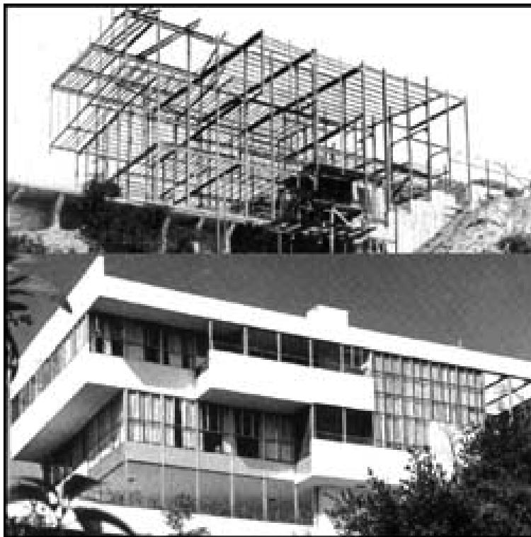
Fig_2.1. 5 : In Lovell's Health House, Neutra explored the industrial nature of production through various means, whereby the atmosphere of the house was created through the considered use of technology. This could be demonstrated by its construction technique, the factory assembled windows and the Ford Model-A headlights installed in the main stairwell. From afar the building seems to be masonry, however it is a lightweight steel frame with gunite (sprayed on concrete).
