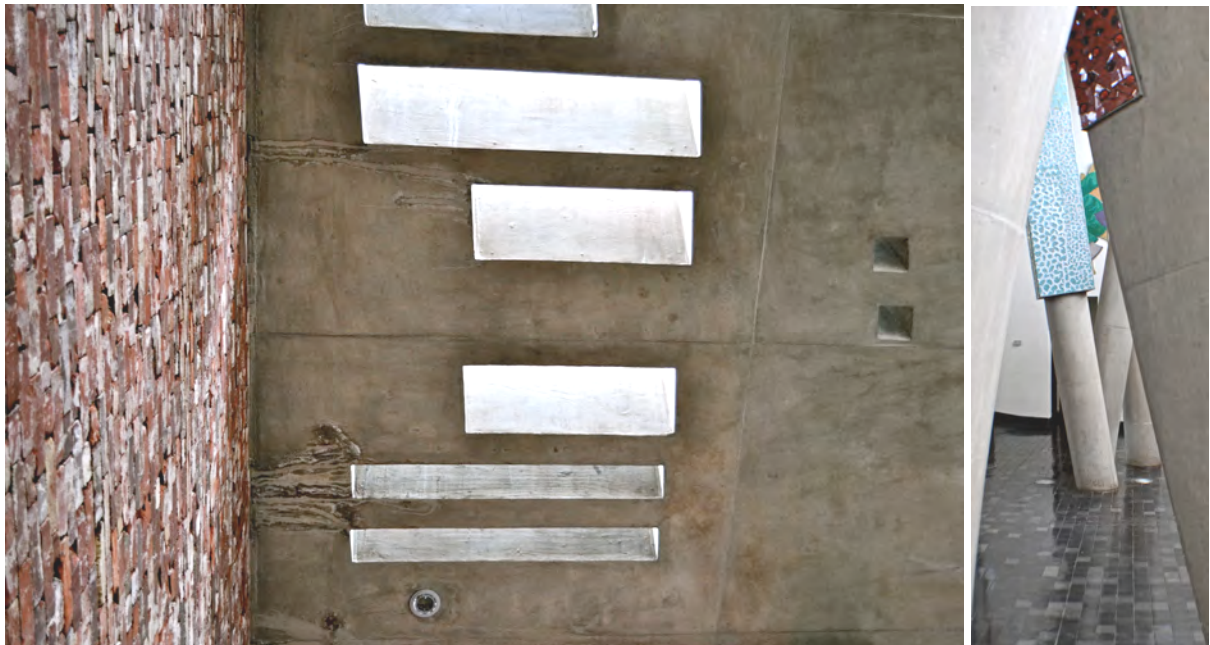
Fig_3.7 : The random roof windows create an abstracted dabbled (north) light which moves through the space. This also shows the primal materiality of the architecture, raw face brick and off-shutter concrete. An awareness to allow the materials to stand for what they are.
