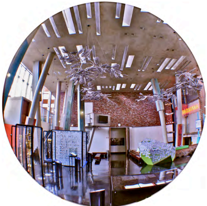
Fig_3. 13 : A view of the foyer, showing the various use of primary, exposed materials; concrete, in the form of tree stump columns and roof canopy, and reclaimed brick from the awaiting trial block.
