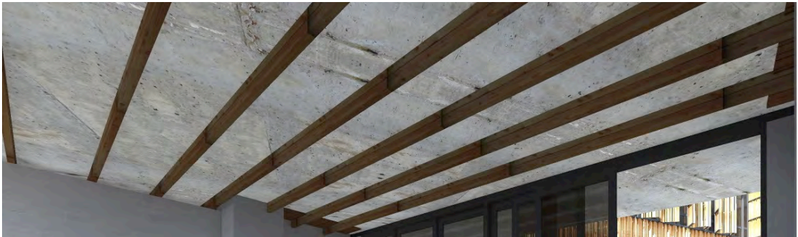
Fig_ii. 28 : Detail of the roof in a typical studio.
