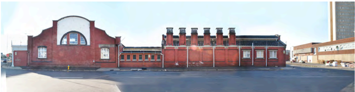
Fig_ii. 4 : South elevation of the beerhall showing the various window treatments.
