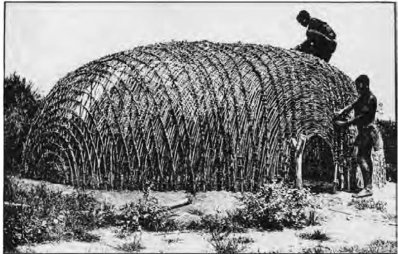
Fig_2.2. 15 : A traditional Zulu beehive hut in Kwa-Zulu Natal, South Africa that directly responds to climate, context. It is resourceful and straightforward to construct and take apart if required to move.
