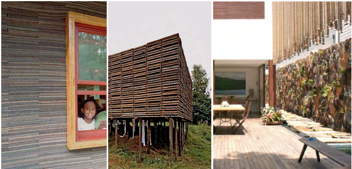
Fig_2.3. 14 : Facades : using recycled carpet tiles. Rural Studio, Carpet tile house, Masons bend, Alabama, USA.
