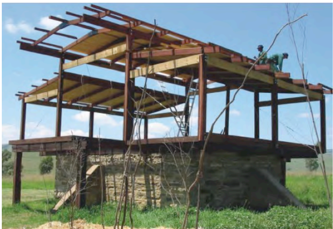
Fig_3. 19 : The reservoir house during construction, demonstrating the relatively simple and robust structural system used.
