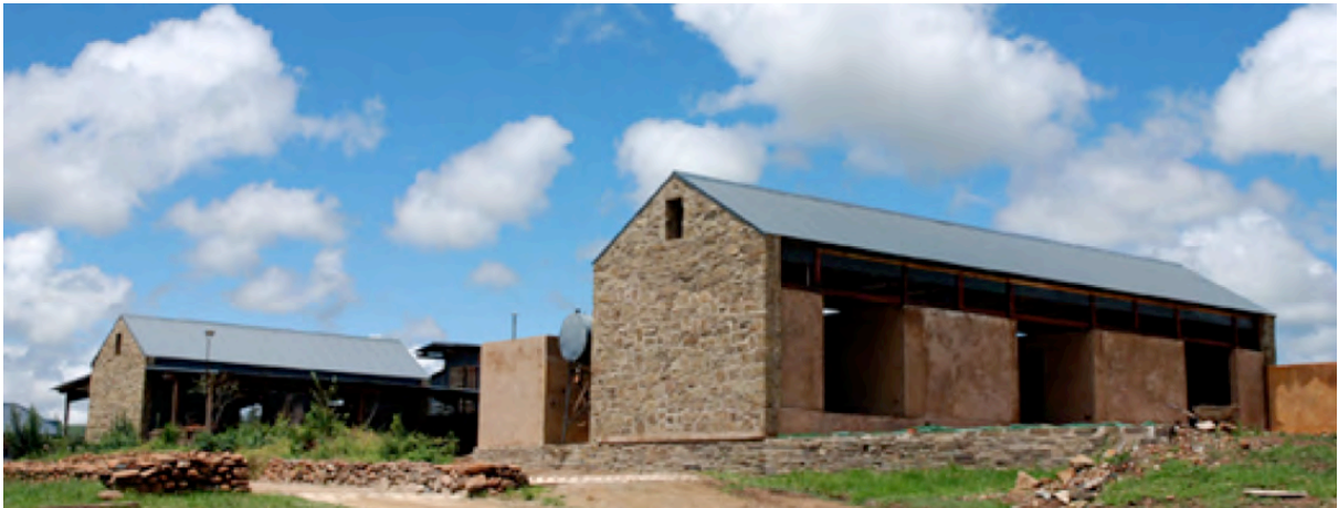
Fig_3. 27 : The workshop, in the process of completion, stands as the workhorse of the development.
