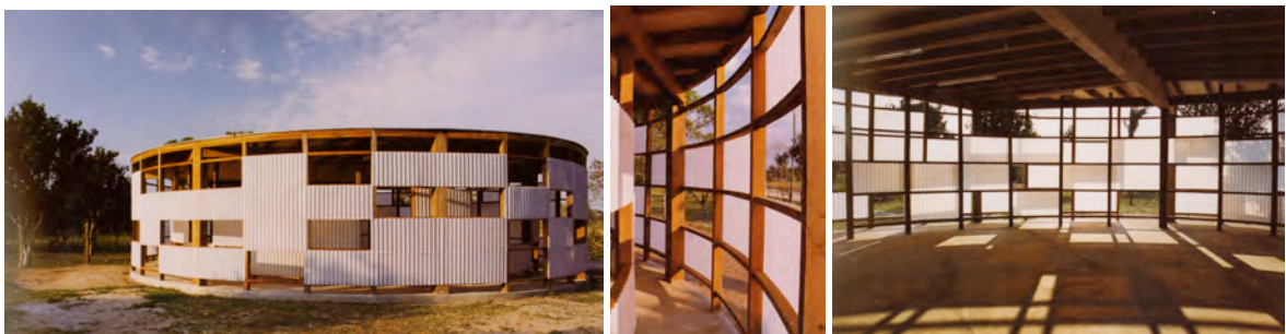
Fig_2.3. 19 : At just over 100sqm, a strong but simple structure encases a flexible public space that has been built with locally sourced timber and various panels of translucent polycarbonate, a relatively inexpensive modern material. This resulted in a construction time of 10 days. Church, Urubo, Bolivia
