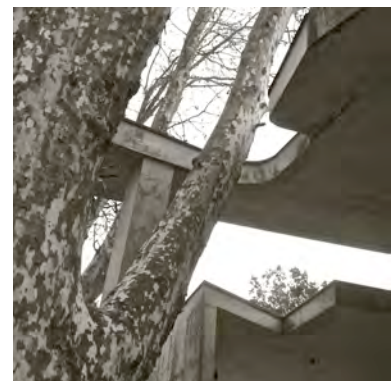
Fig_4.3 : The architects carefully wrapped the roof slabs around the existing trees. A direct response to the peculiarities of the site. Electric Ladyland roof detail, Kloof, Durban.
