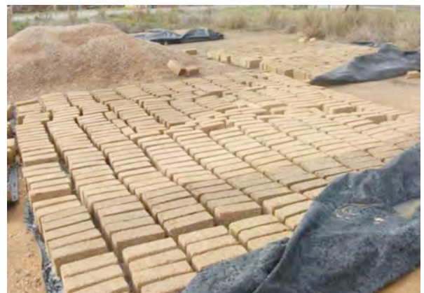
Fig_2.2. 17 & Fig_2.2. 18 : A sustainable hand-made building material, hand made on site using local sand and 5% cement/concrete stabiliser : Job creation, low carbon footprint, fire resistant, and creates a recyclable building material with no pollution.
