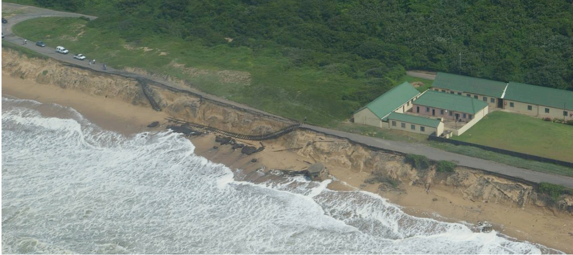
Figure 9.5: Erosion along the base of the Bluff from the 2007 storm showing the undermining of the old rail line along the toe of the Bluff and the current access road. (Photo: A. Mather).
