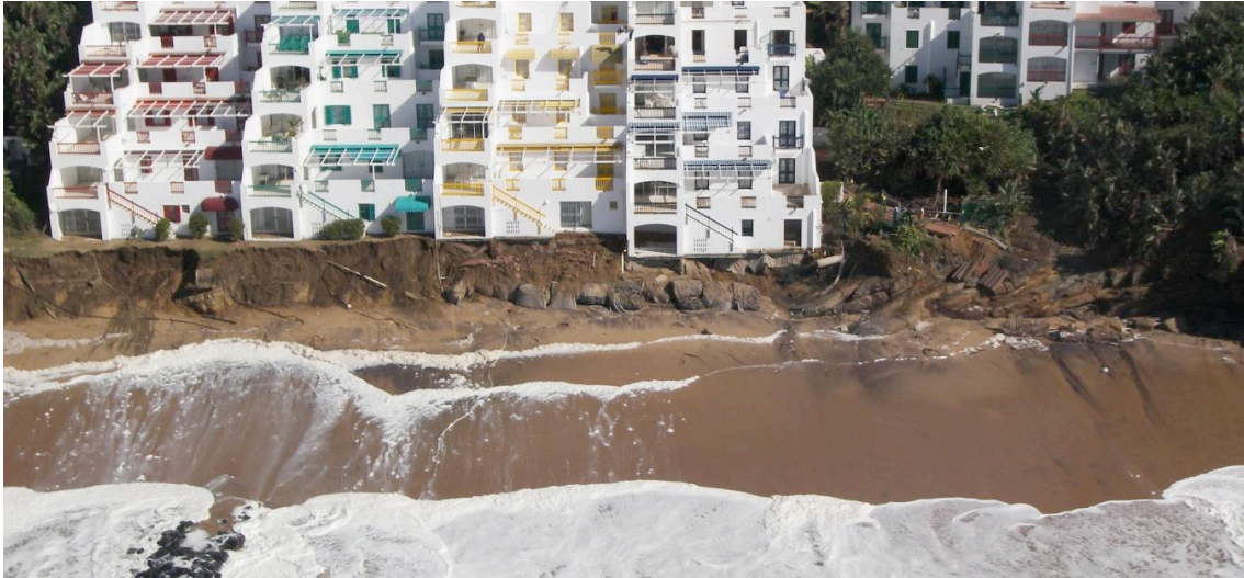
Figure 9.3: Santorini complex showing infilling and exposed sea protection works. Location approximately 20 kms north of Durban. (Photo: S. Bundy).
