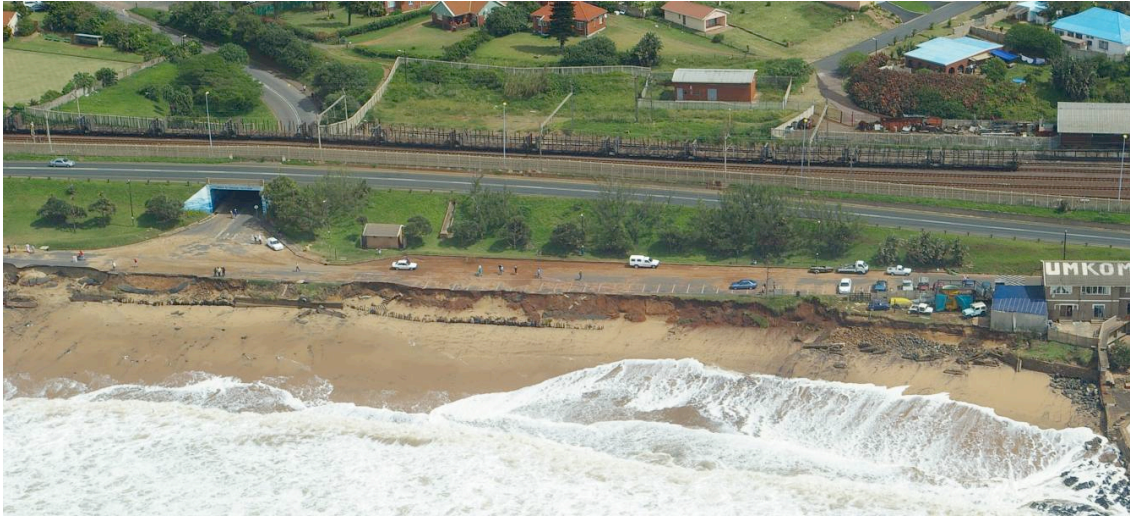
Figure 9.4: Erosion at Umkomaas from the 2007 storm showing the erosion of the previous sea defense, carpark and access road. (Photo: A. Mather).
