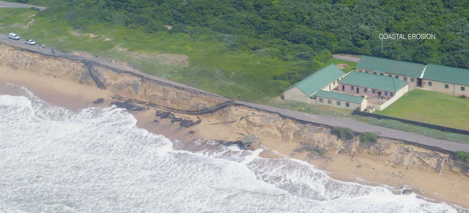
Figure 5: Erosion along the base of The Bluff (Photo: A Mather)
