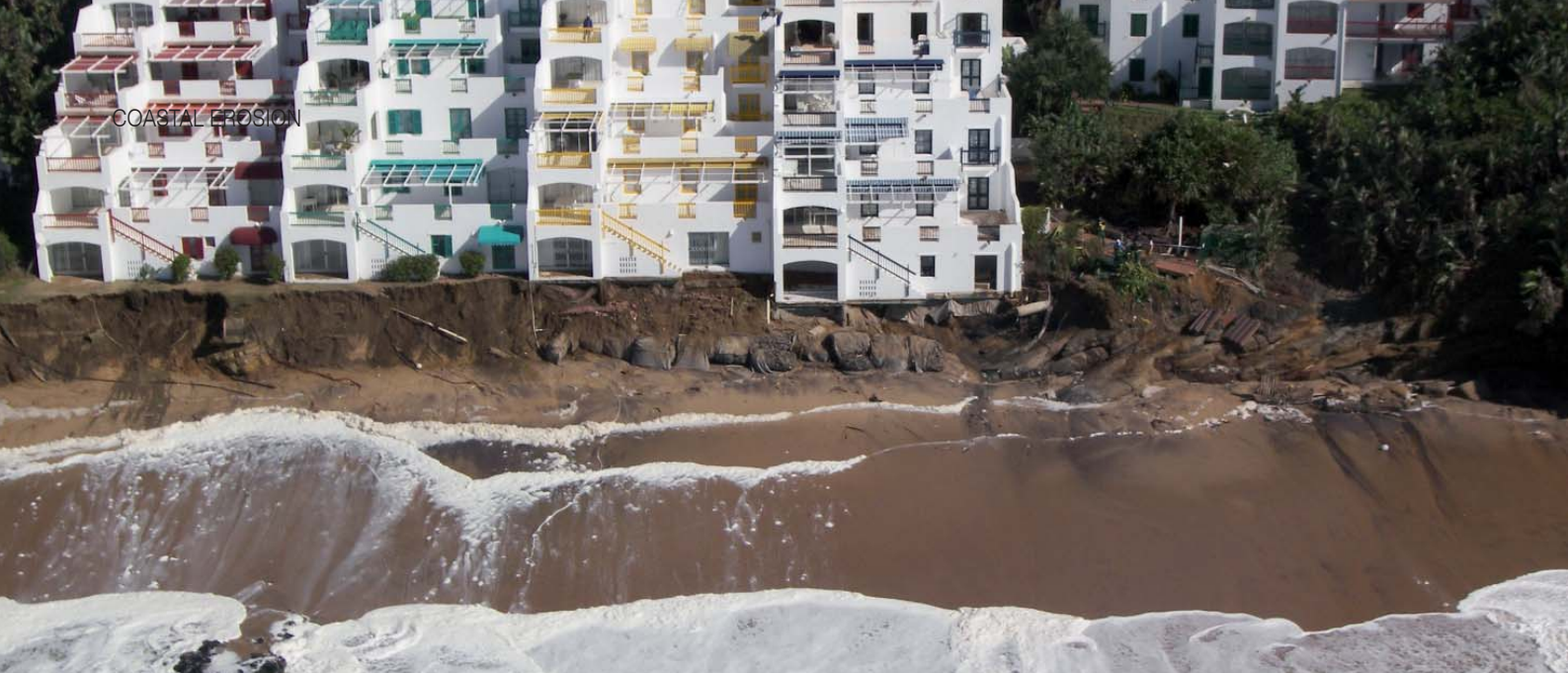
Figure 3: Santorini complex showing infilling and exposed sea protection works
