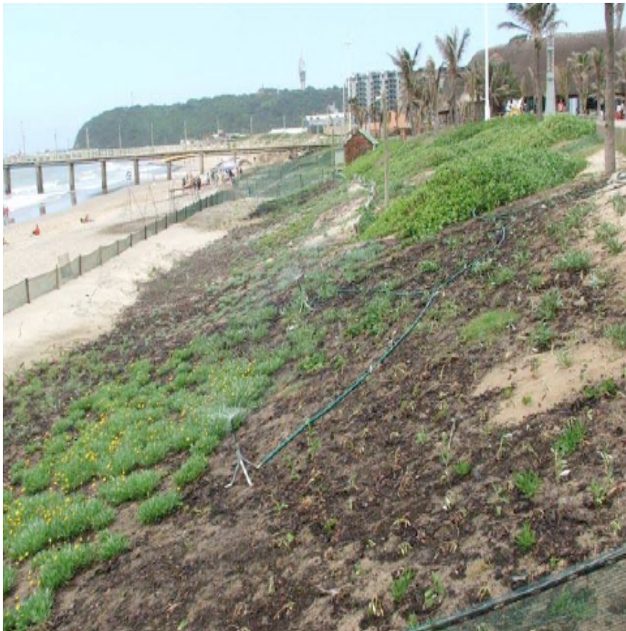
Figure 10.9: Dune re-establishment in front of Ushaka Marine World at the Point (Photo: M Pauselli).
