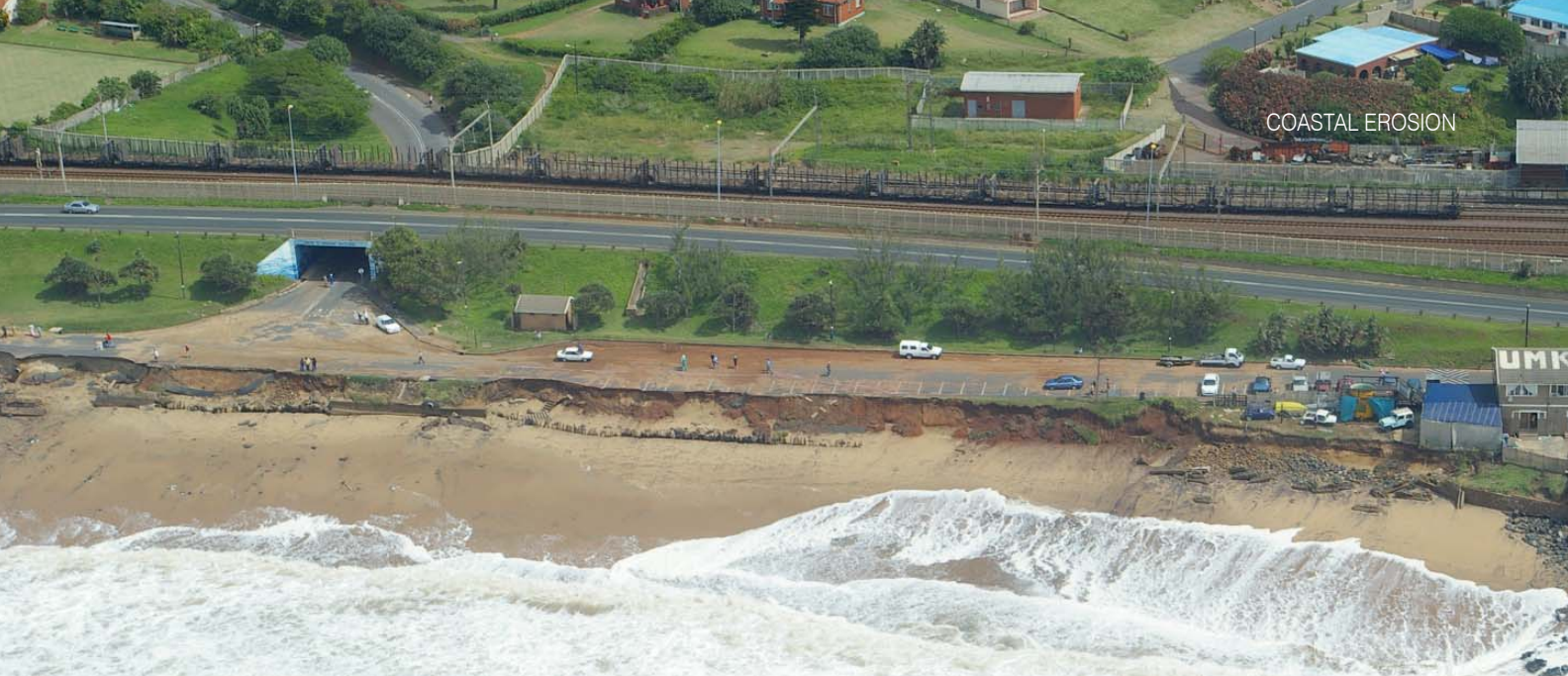
Figure 4: Erosion at Umkomaas
