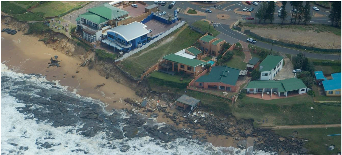
Figure 9.6: Erosion in Ballito from the 2007 storm showing the damaged beach facilities/toilet block and loss of sediment from this beach. (Photo: A. Mather).
