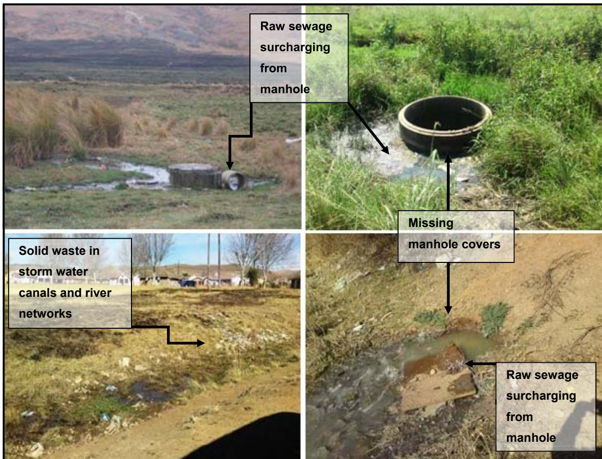
Figure 3.4: Observed potential water quality impacts in Mpopomeni settlement
