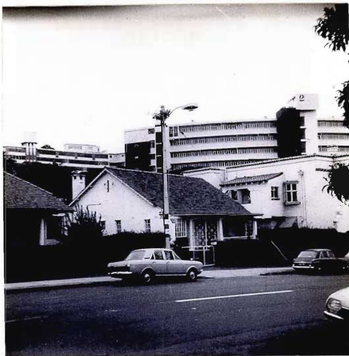
A group of slab blocks in Musgrave Road blocking off the view from those buildings behind them.
