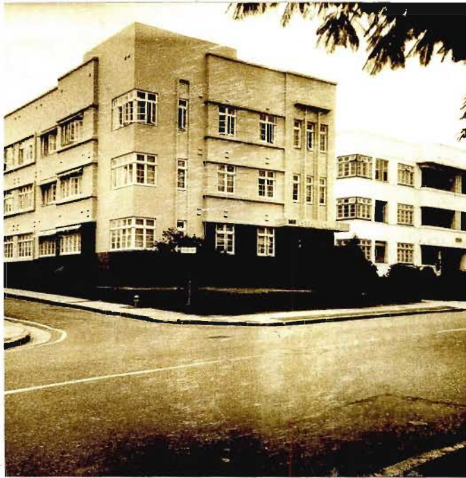
A typical 3-storey block built close to the building line.
