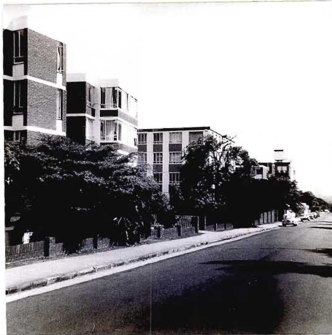
Another view of the typical development taking place on the Low Berea.
