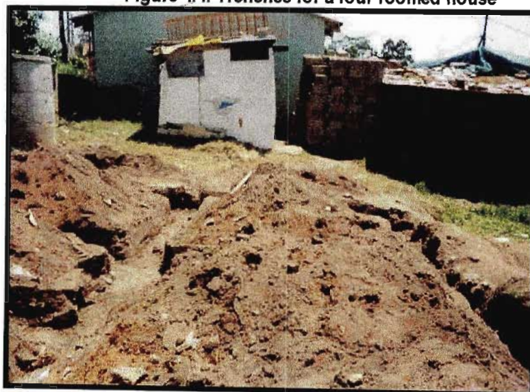
Figure 4.4: Trenches for a four roomed house
