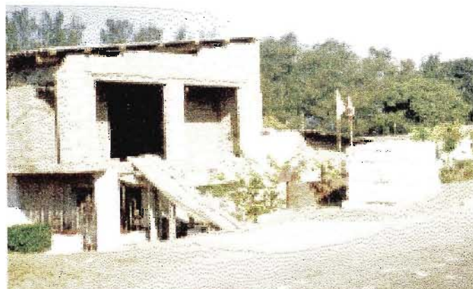
Plate 16: A Residence in Merewent, undergoing extension – demonstrating one facet of resident's investment into the place
