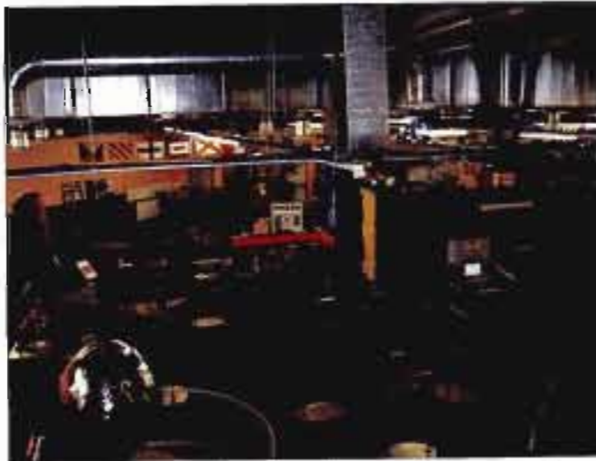
Fig 4.18: The overhead services are left exposed (Source: author)
