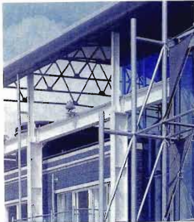
Fig 3.28: The existing façade is revealed and the added space frame further enhances the technical feel of the building. (Source: Hall, 1995: 38)
