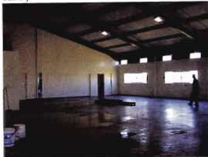
Fig 4.5: The new exhibition space with day lighting and power supplied from below. (source: author)
