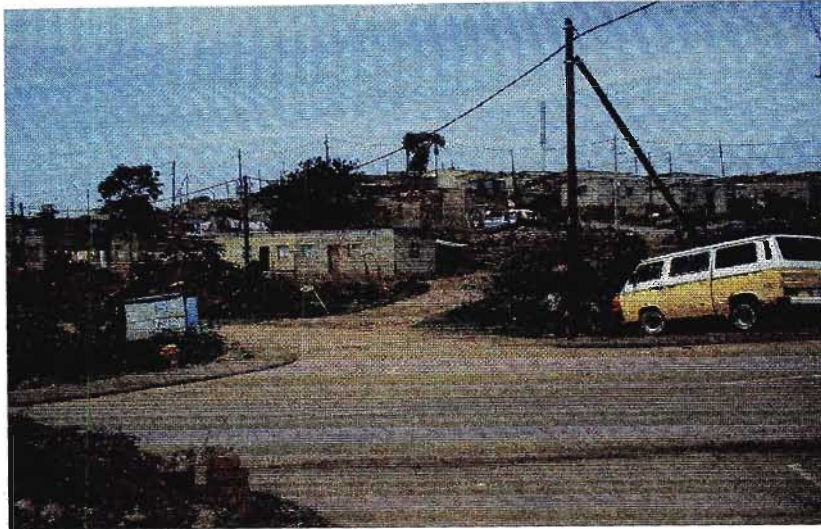
Figure 4.1: Part of Wiggins uMkhumbane low cost housing project
