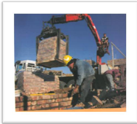
Figure 4-7 Construction worker on the job
