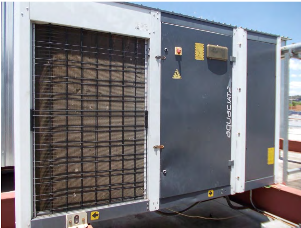
Figure 7.1: Mechanical Compression Chiller at the Moot Hospital Plant
