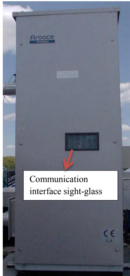
Figure 7.16: 35kW Absorption Chiller on the roof of Netcare's Moot Hospital in Pretoria
