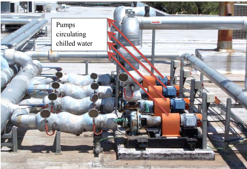
Figure 7.4 Pumps circulating chilled water between the buffer tank and air handler
