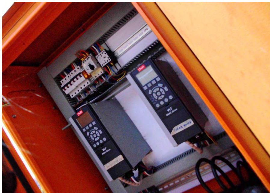
Figure 6.4: Solar irradiation data was logged and stored for retrieval on a memory card in this panel
