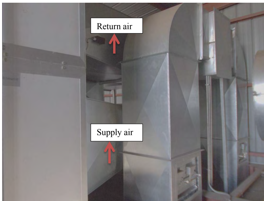
Figure 7.11: Supply and return air ducting
