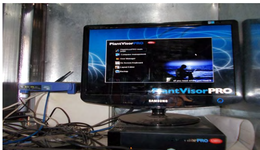
Figure 6.2: BMS System Computer programmed through PlantVisorPro software
