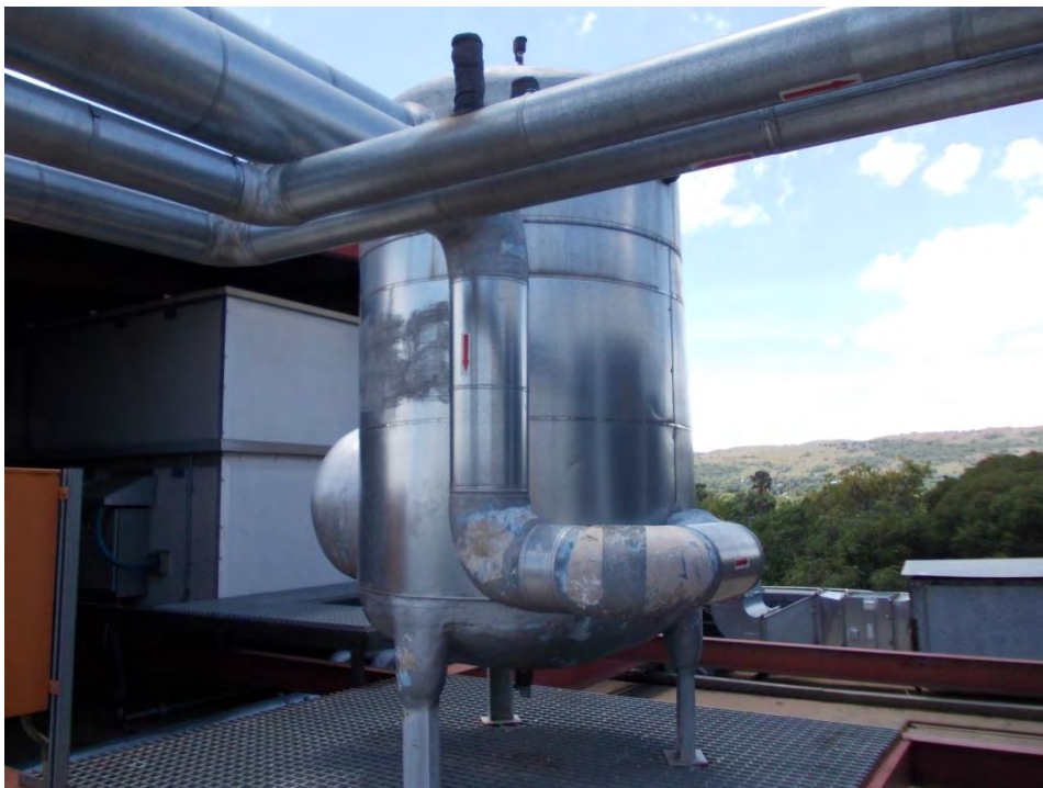
Figure 7.2: Chilled water buffer tank to which chilled water is sent from the chiller
