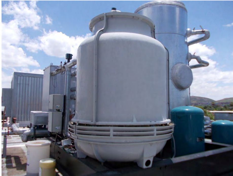
Figure 7.24: Cooling Tower (in front)
