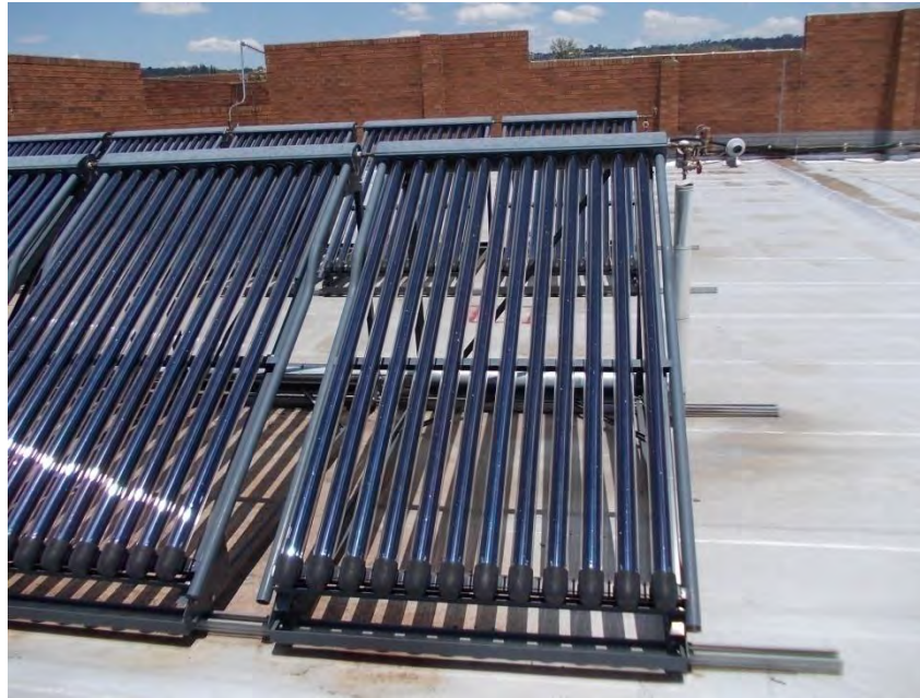
Figure 7.13: Heat pipe Solar Collectors on the roof of Netcare’s Moot Hospital in Pretoria
