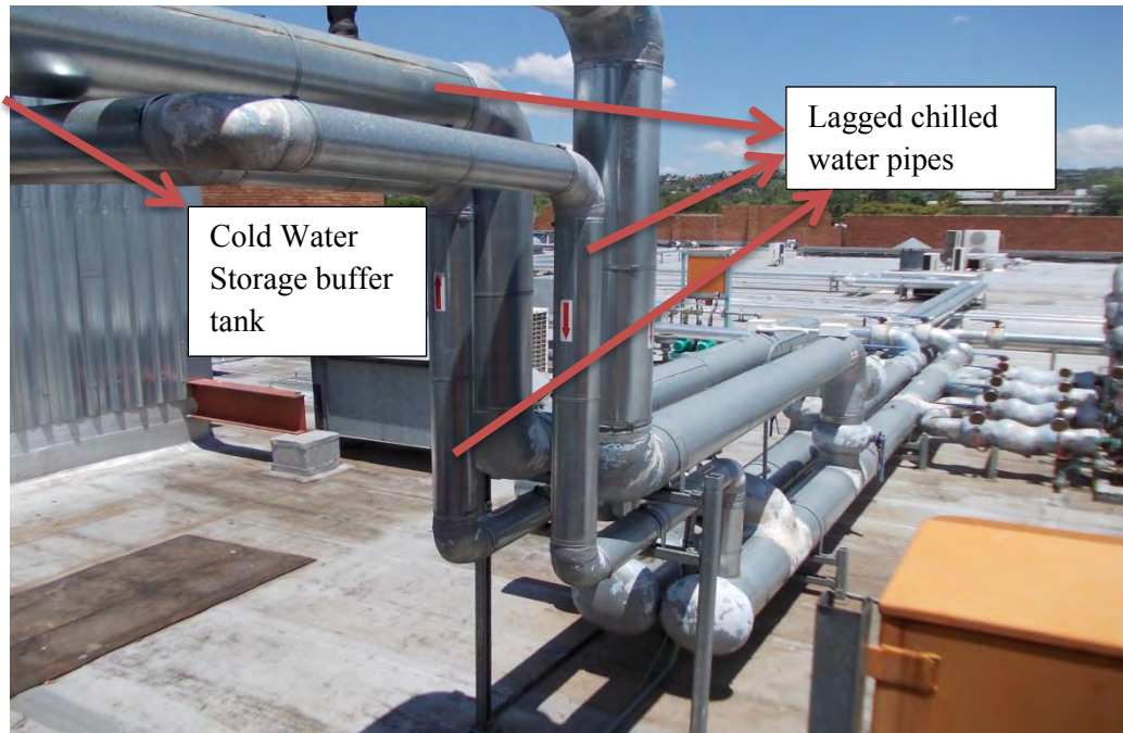
Figure 7.3 Lagged Chilled Water Pipes leading from buffer tank (top left) to pumps
