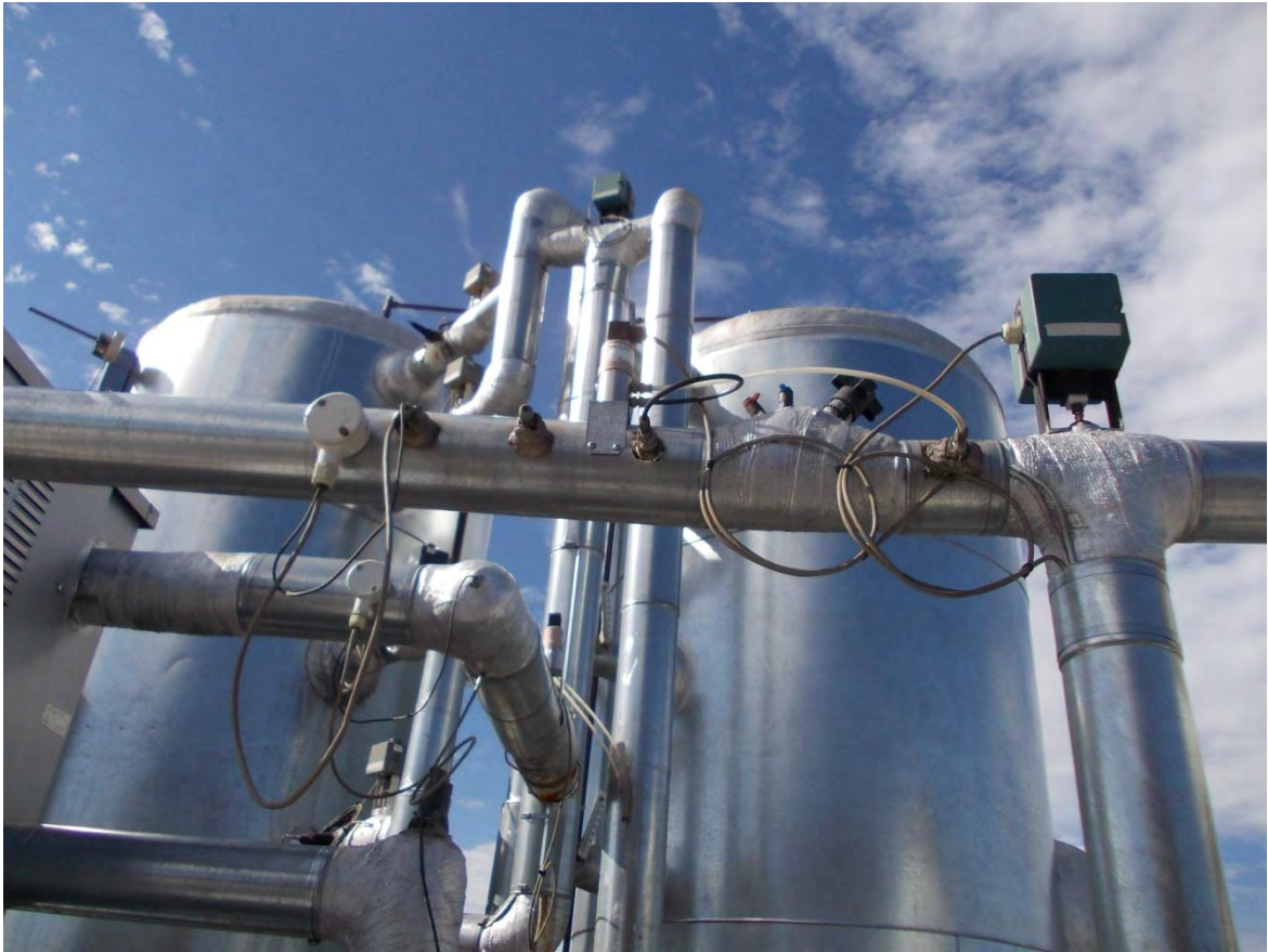
Figure 6.7: Temperature probes on a section of the absorption cooling system
