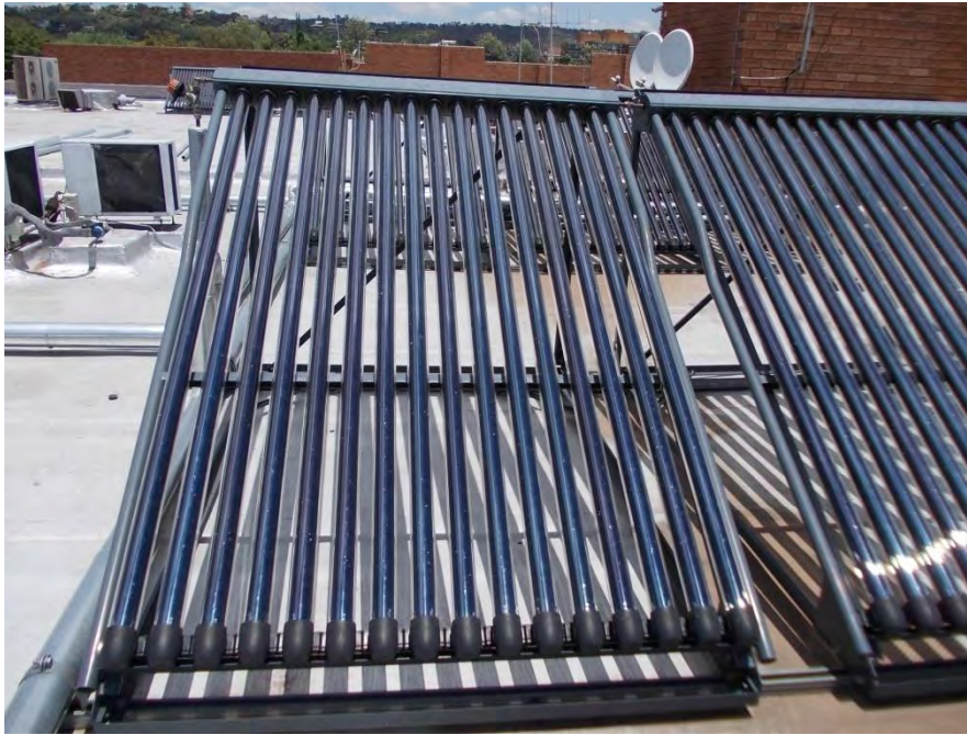
Figure 7.12: U-pipe Solar Collectors on the roof of Netcare’s Moot Hospital in Pretoria
