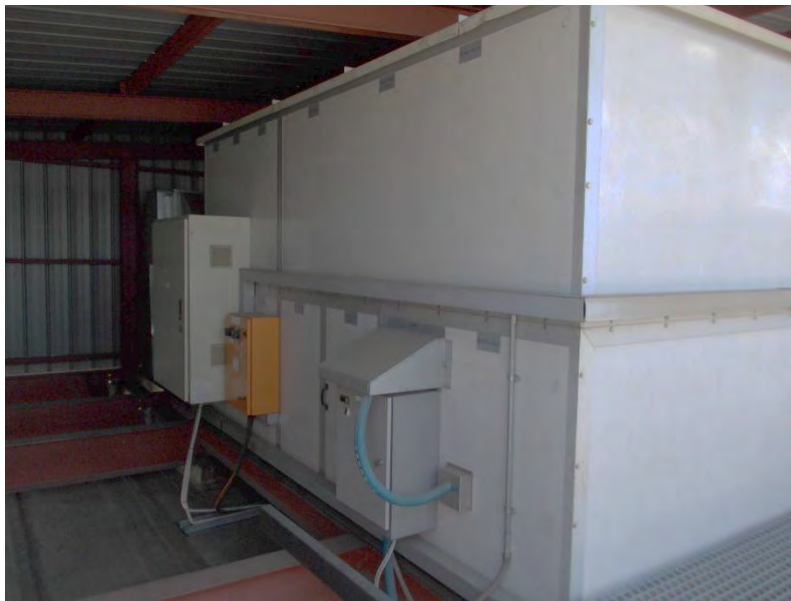
Figure 7.5: Air handling unit
