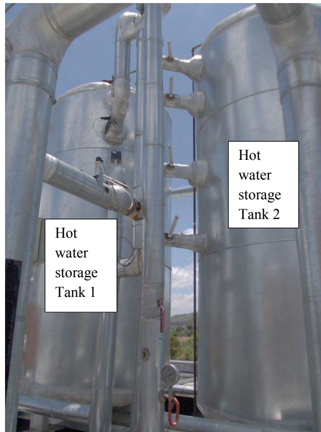
Figure 7.14: Two 6000l hot water buffer tanks
