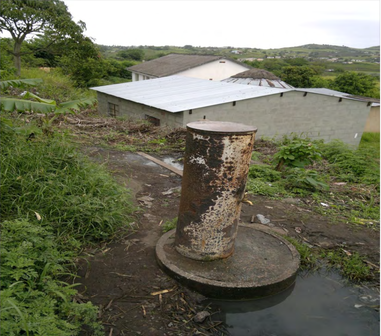
The type of standpipe existed in the past: A photograph taken by Mlethwa at eMahlongwa.
