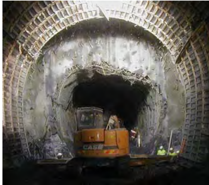
FIGURE 2-1 - SAINT MARTIN LA PORTE ACCESS ADIT AT CHAINAGE 1325 M BEFORE RE-SHAPING THE TUNNEL CROSS SECTION (BARLA, BONINI, DEBERNARDI, (2010))
