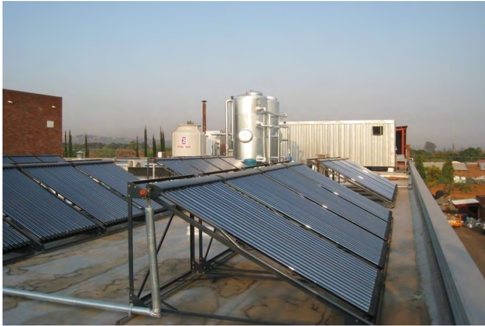
Figure 5.4: Photograph of the arrangement of the Solar Collector Array
