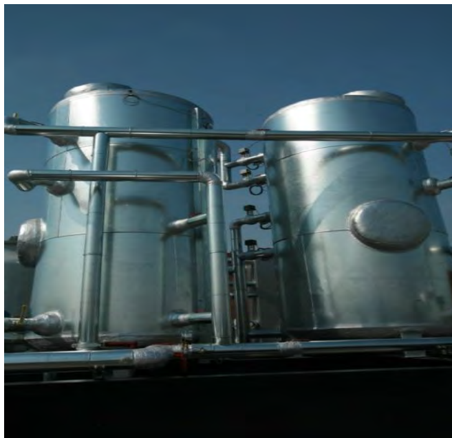
Figure 5.5: Photograph of the two hot water storage tanks
