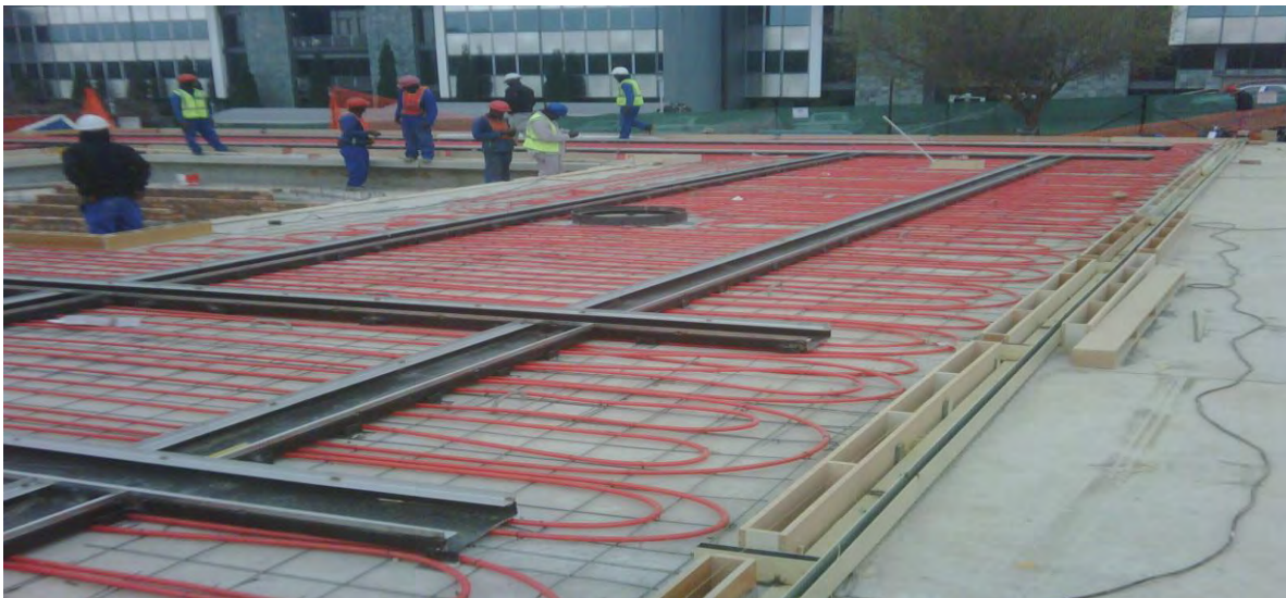
Figure 5.11: Photograph of the thermally active slab under construction
