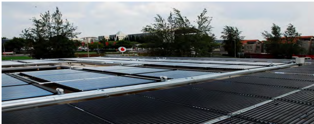
Figure 5.10: Photo of the Solar Collector Array at Vodafone SSIC
