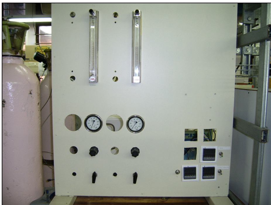
Fig J: Control board containing various components (pressure regulators, rotameters, pressure gauges, temperature controllers).
