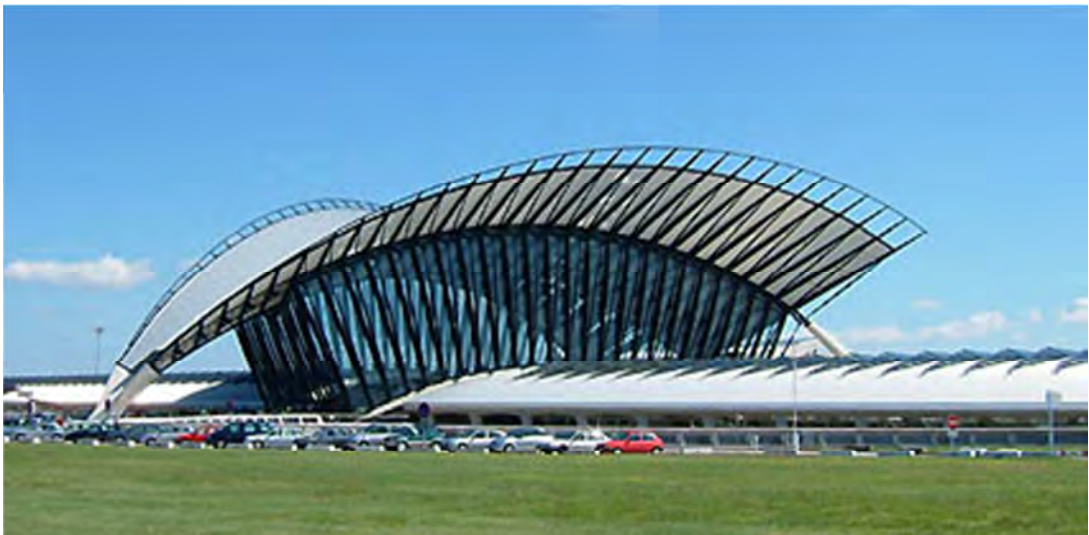
Plate 39: Main Arch Photograph (Glynn, 2004)
