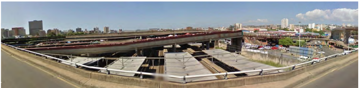
Plate 76: Bereja Station Platforms from Canongate Road
