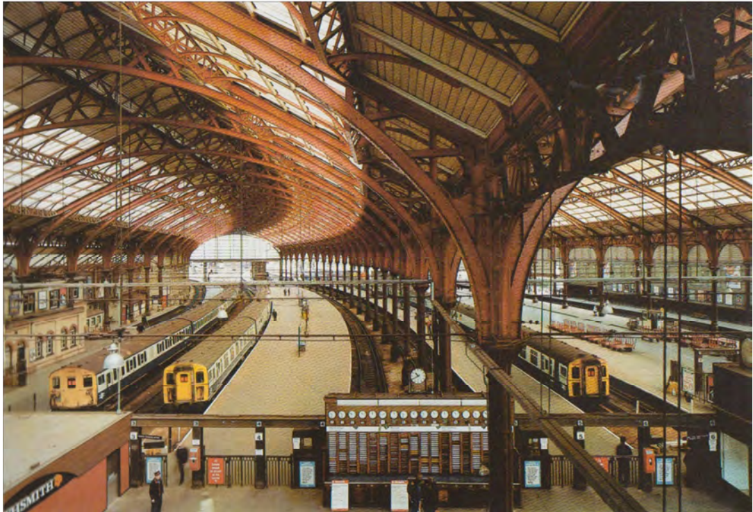
Plate 53: Brighton Station (Hamm 1984)
