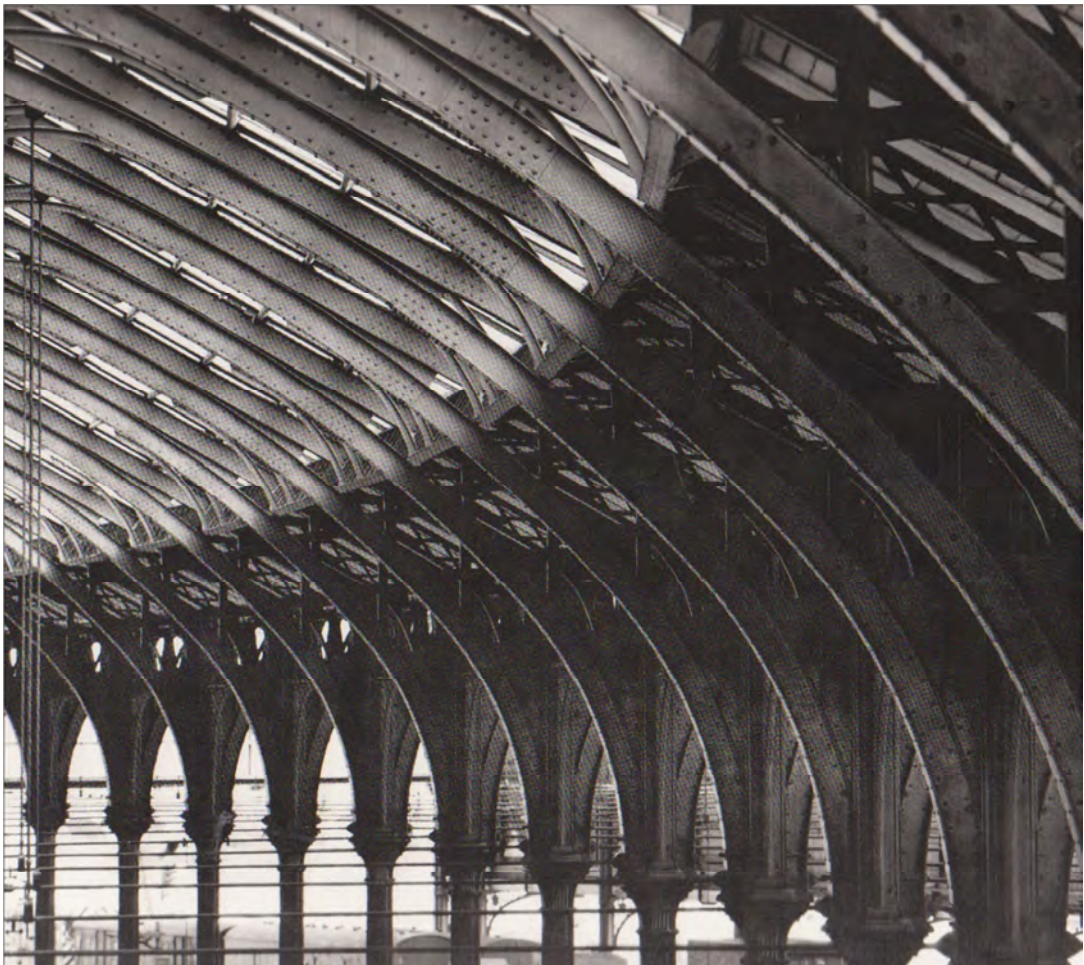
Plate 54: Brighton Station (Hamm 1984)
