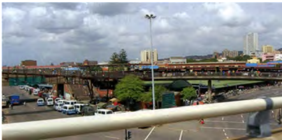
Plate 16: Pedestrian Bridges (Dobson, 2001)
