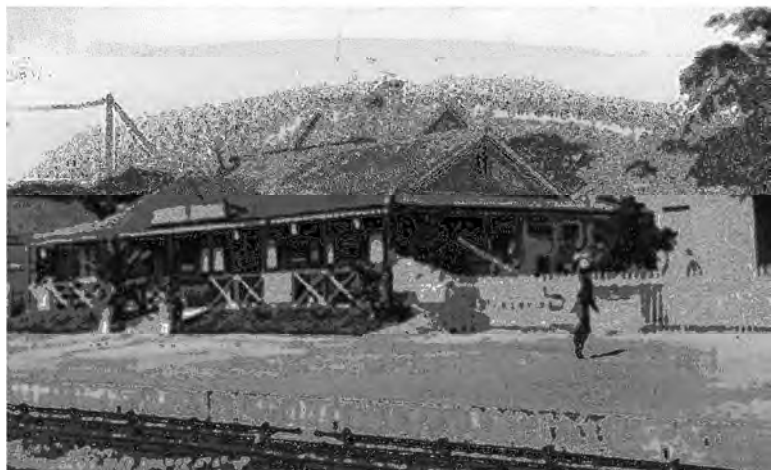
Plate 77: Old Bereja Station form Opposite Platform
