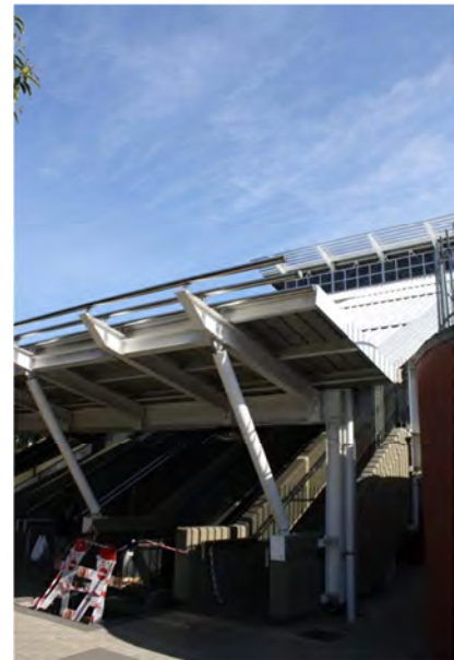
Plate 61: Station Entrance / Rail
