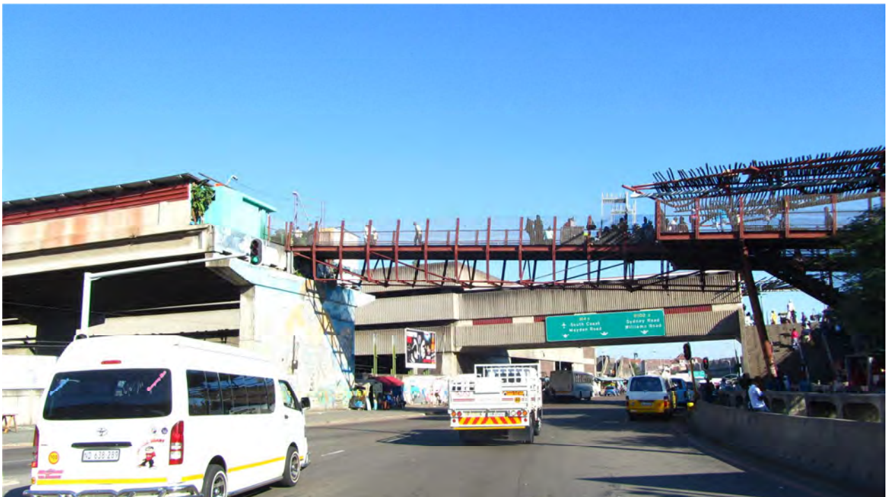
Plate 90: Berea Station from Market Road
