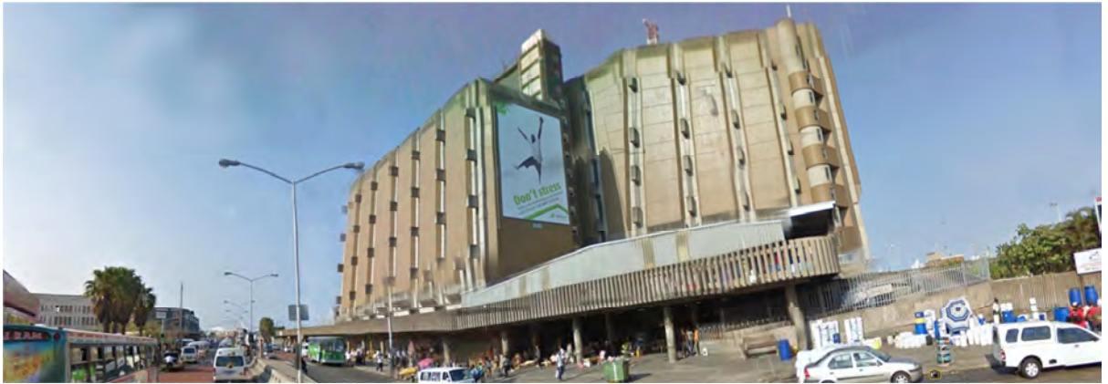
Plate 9: Image B, Durban Station - Umgeni Road (Google Earth, 2010)
