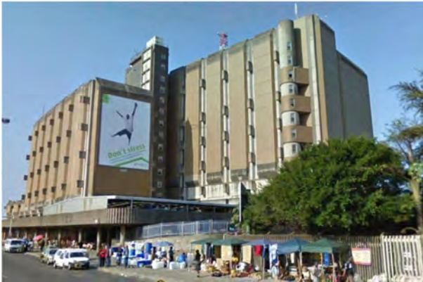
Plate 66: Umgeni Road Entrance and Office Block
