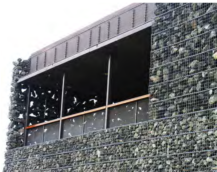
Dominus Winery - Herzog & de Meuron Plate 9.3 - Lightweight steel construction used on the upper floor.
