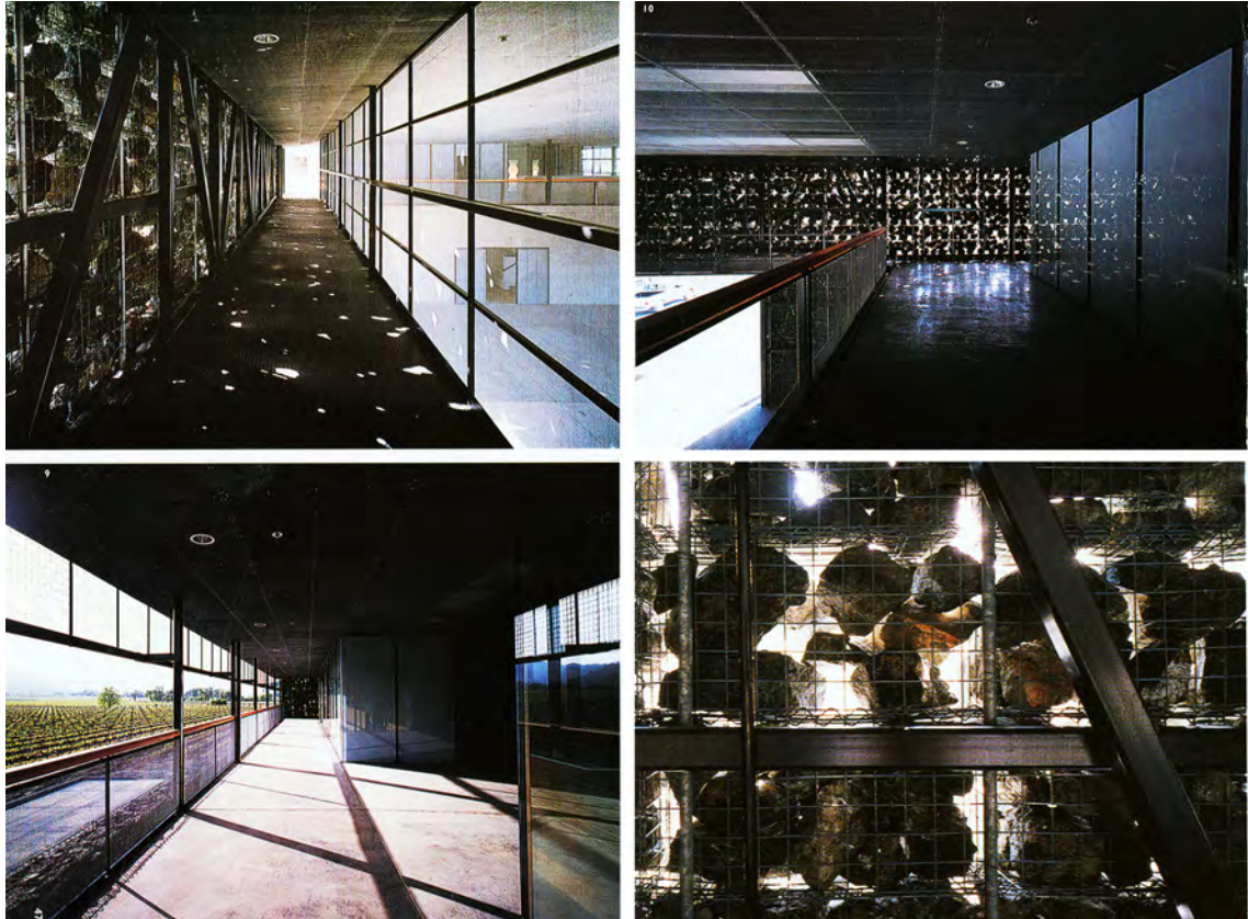
Dominus Winery - Herzog and de Meuron Plate 3.14 (above left and right) - kinetic use of light and shadow as a result of stone wall. Plate 3.15 (below left) - corridor space open to environmental phenomena. Plate 3.16 (below right) - construction of basalt stone wall.
