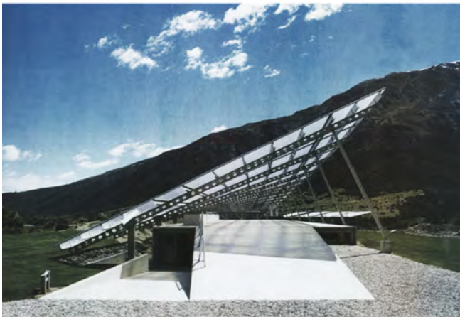
Peregrine Winery - Architecture Workshop Plate 9.8 - The simplistic form of the Peregrine Winery.
