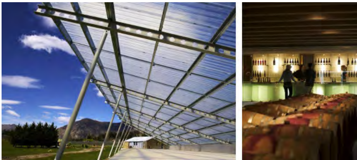
Peregrine Winery - Architecture Workshop Plate 9.9 (left) - Steel and Durolite roof construction. Plate 9.10 (right) - The tasting room.
