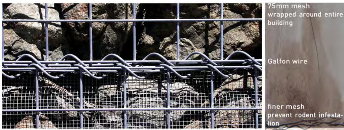
Dominus Winery - Herzog & de Meuron Plate 9.2 - Basal stone wall construction showing wire mesh and the Galfon wire.
