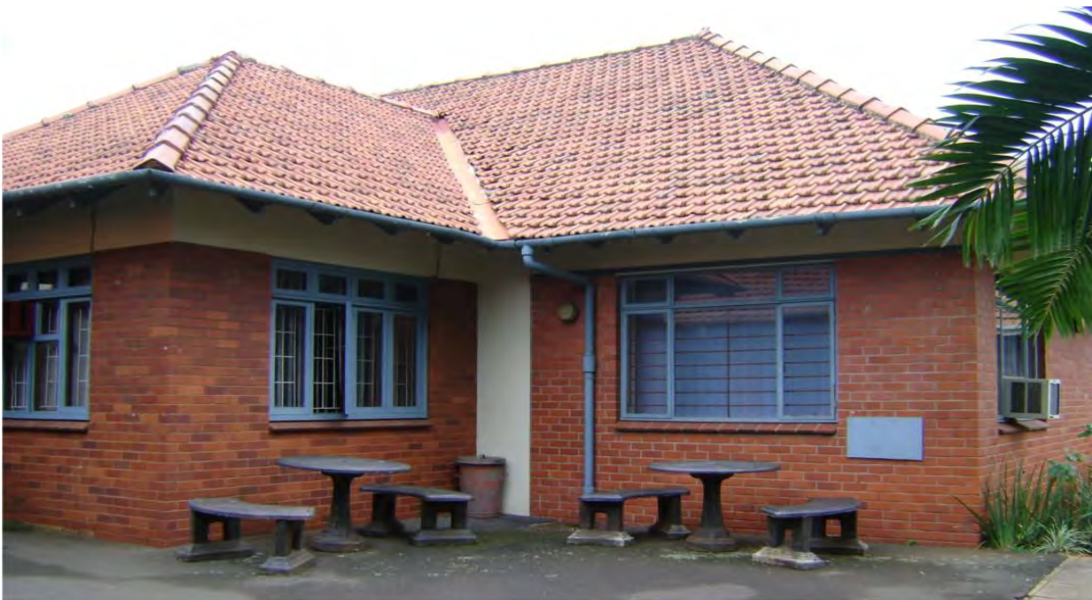
Plate 7.16: The architectural expression of the school which resembles the surrounding residential architecture of the suburb of Glenwood (Source: Author).
