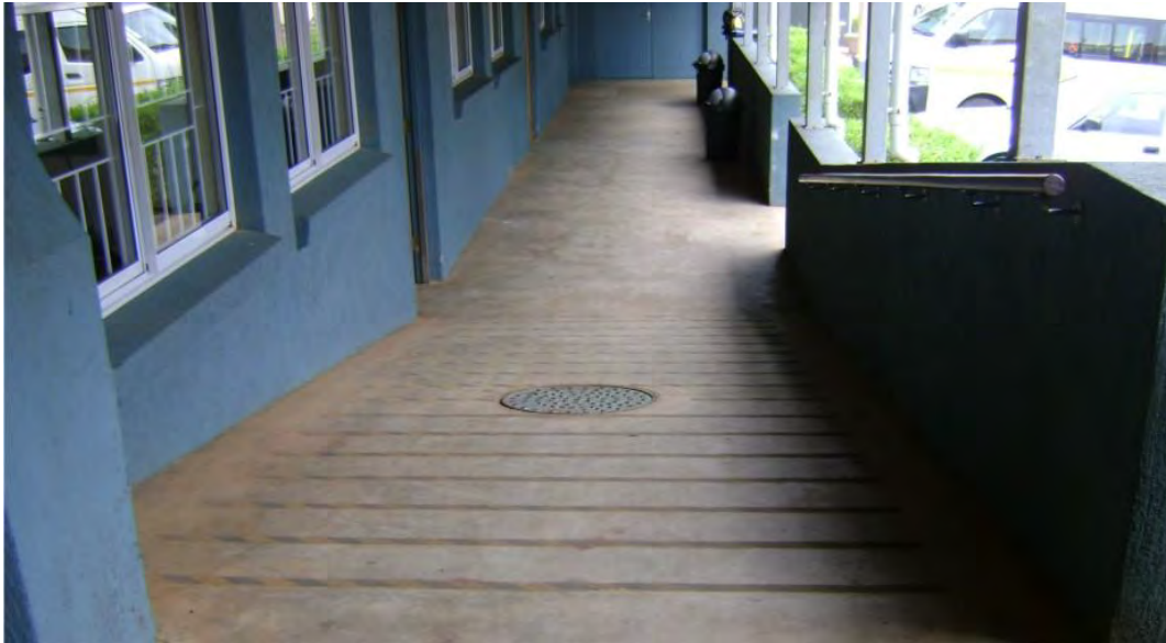
Plate 7.13: A ramp at the school (Source: Author).
