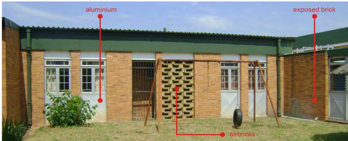
Plate 7.10: An elevation showing the use of different textures (Source: Author).
