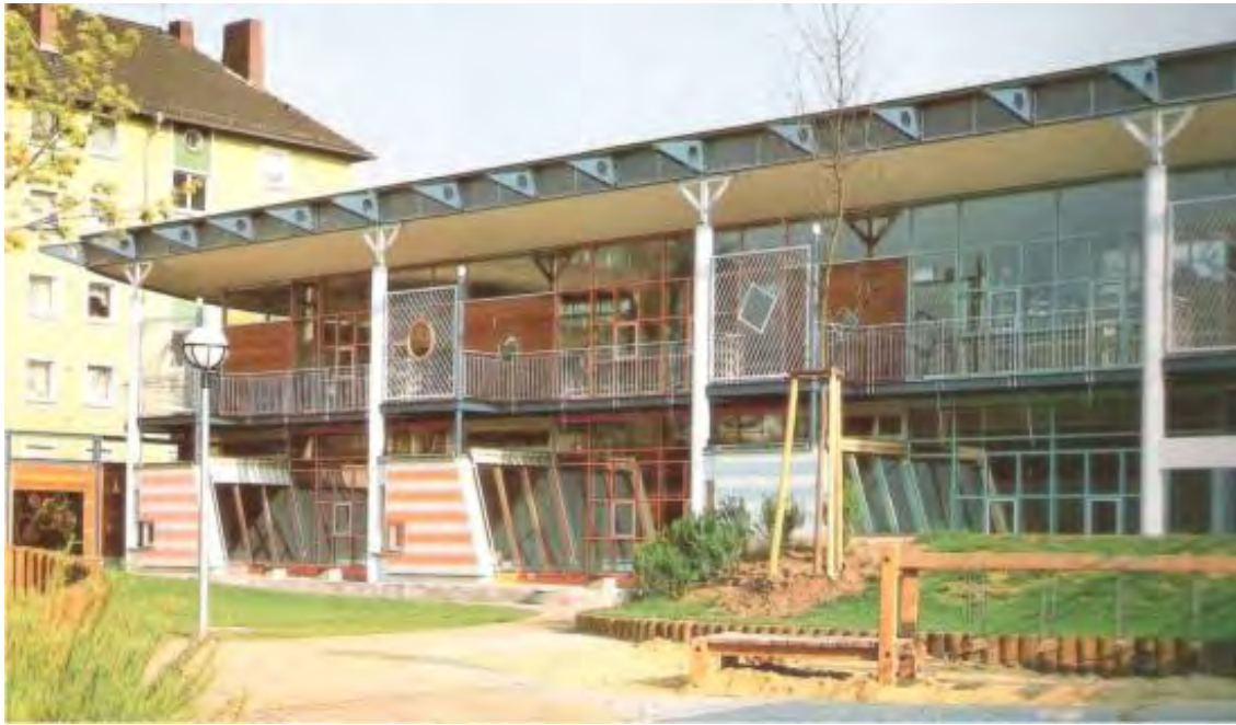
Plate 4.6: Buildings can be designed to entice all of our sensory systems, such as this school which incorporates textures, patterns, shapes and planting to appeal to one's visual and tactile senses (Kroner, 1994: 18).
