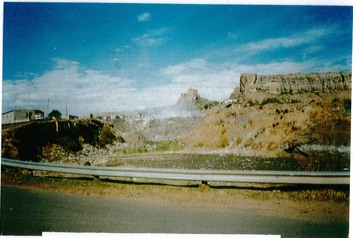
(Pic-2) Leachate at Ts`osane dump-site. Does the law care if it reaches the not so far away Maqalika dam?
