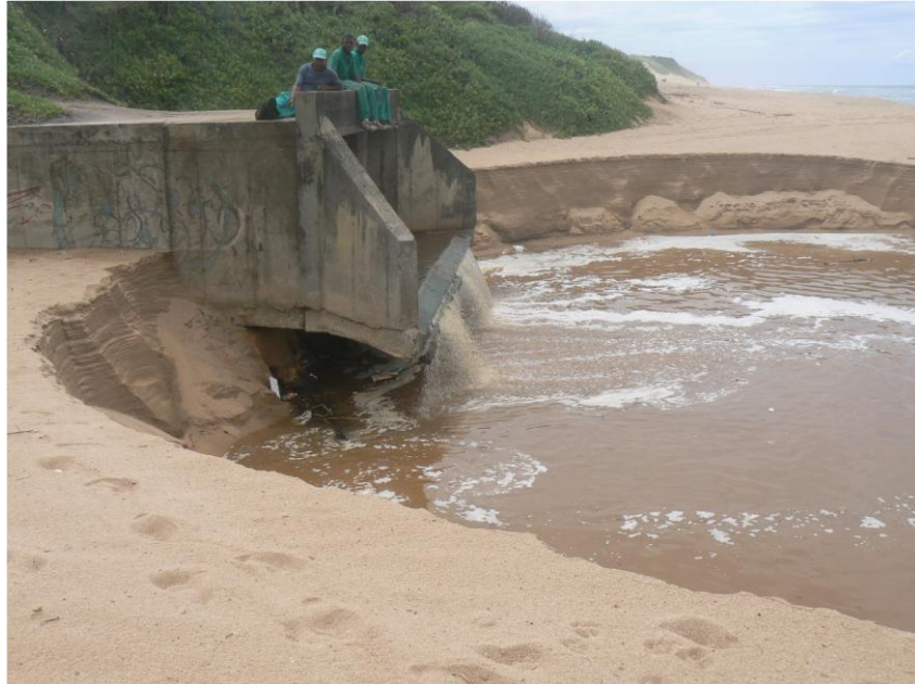
Figure 4.5. Numerous storm- and wastewater outlets are scattered along Durban beaches. These hard structures not only release vast amounts of pollutants onto beaches, with potential detrimental effects to sandy beach organisms, but also promote beach erosion (Photo: L. Harris)
