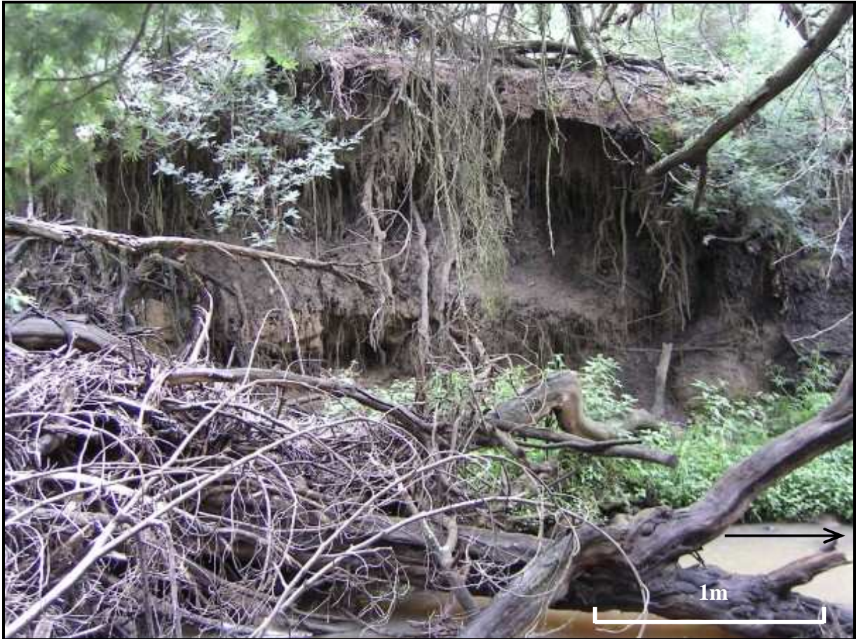
Figure 7.18 Left bank of transect 3 at IAP infested Site C1
