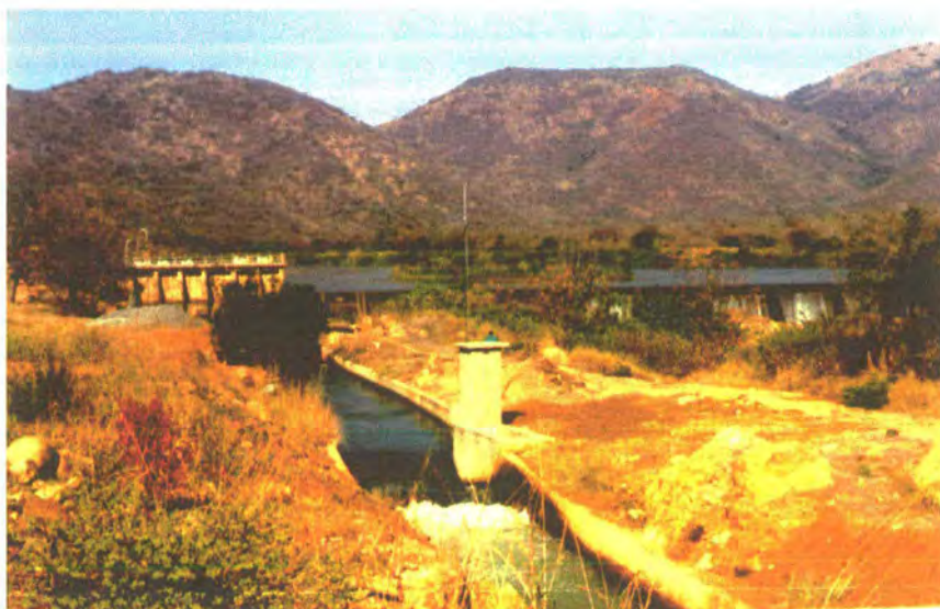
Figure 5.12 Photograph of Grootdraai weir and the main irrigation canal
