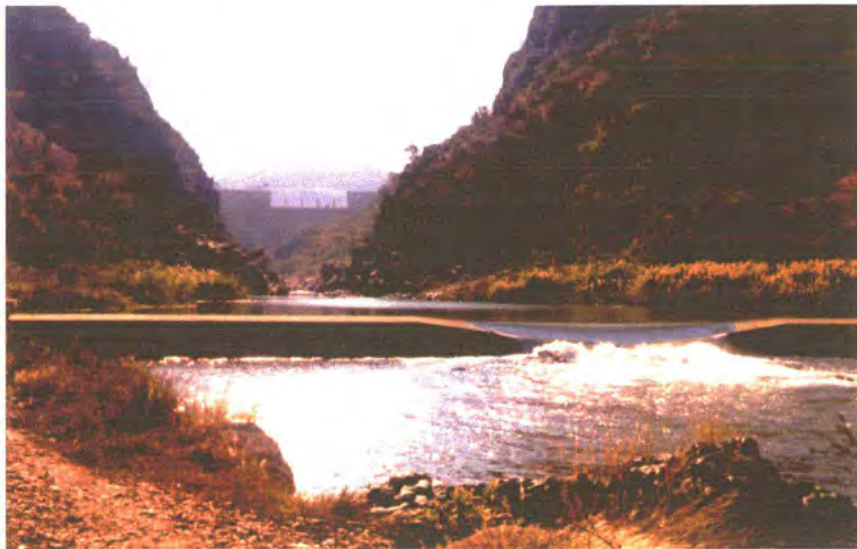
Figure 5.11 Photograph of the measuring weir below the Paris Dam wall
