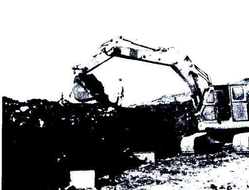
Plate 4.11 Excavator placing Pine-Bark cover on Windrow 1
