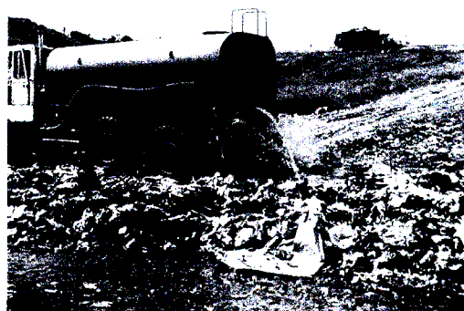
Plate 4.8 The water truck passed over the waste during the construction of Windrow 2
