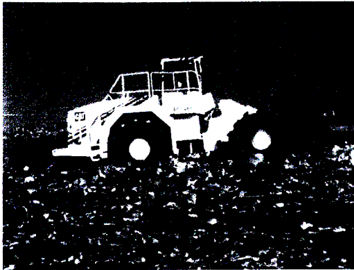
Plate 4.3 Landfill compactor shredding/crushing the waste
