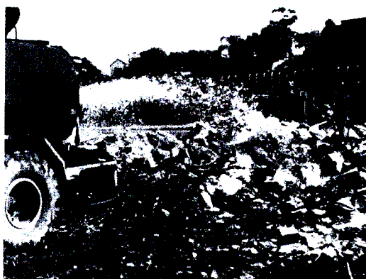
Plate 4.7 Water Truck Spraying water onto waste stockpile during the construction of Windrow 1
