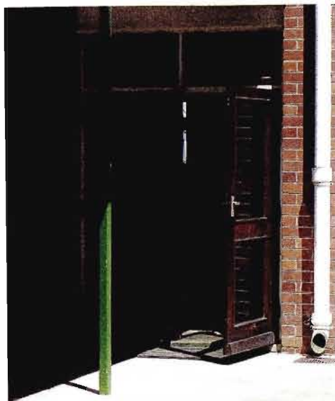
III 5.40: Example of a pole situated in front of a door
