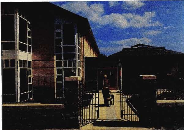
Ill 4.15: Street Entrance (Dawson: 1993,41)
