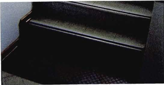
III 5.20: Tactile markers at base of stairs
