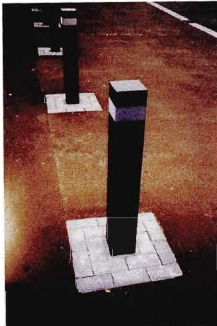
Ill 3.2: change of texture surrounding bollards warns of potential hazard (Barker: 1995,44)
