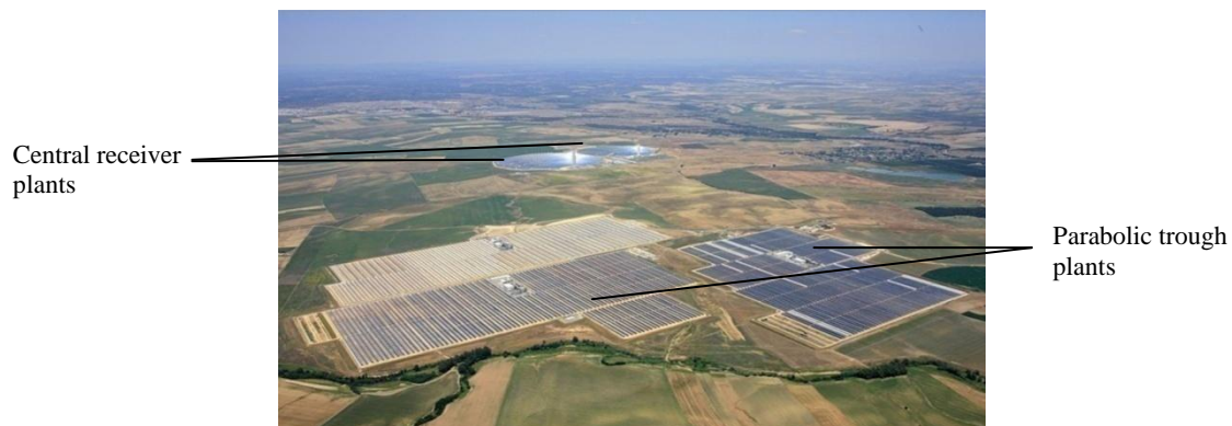
Figure 2.2 Aerial view of the Solucar Platform in Seville, Spain, showing the Solnova solar power plant using parabolic trough technology and the two central receiver plants, PS10 and PS20 for electricity generation (Abengoa solar, 2011).
