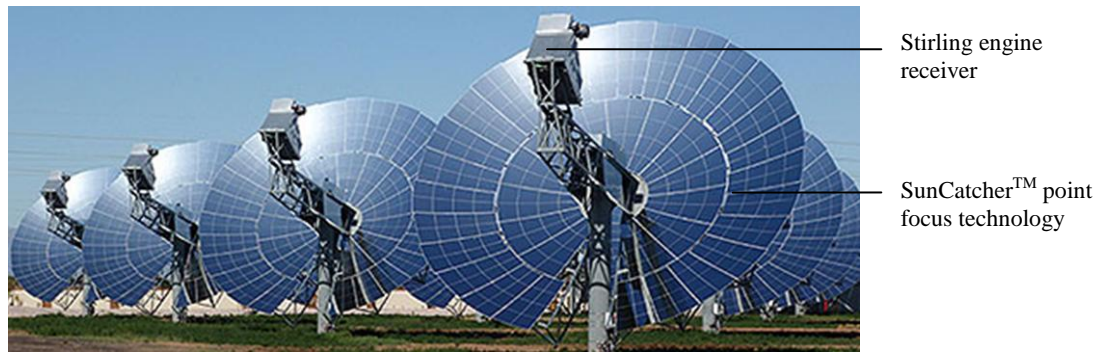
Figure 2.3 Maricopa solar thermal plant in Arizona, USA. The CSP plant houses sixty SunCatcher™ dishes, each with a power rating of 25 kW (Power technology, 2011).
