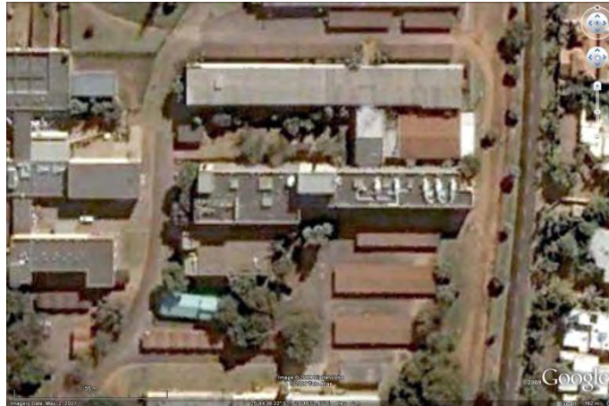
Figure 7.13: CSIR Building 14F & 14E, Source: Google Earth
