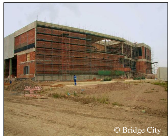
Plate 9.3: Construction of the Bridge City Mall.
