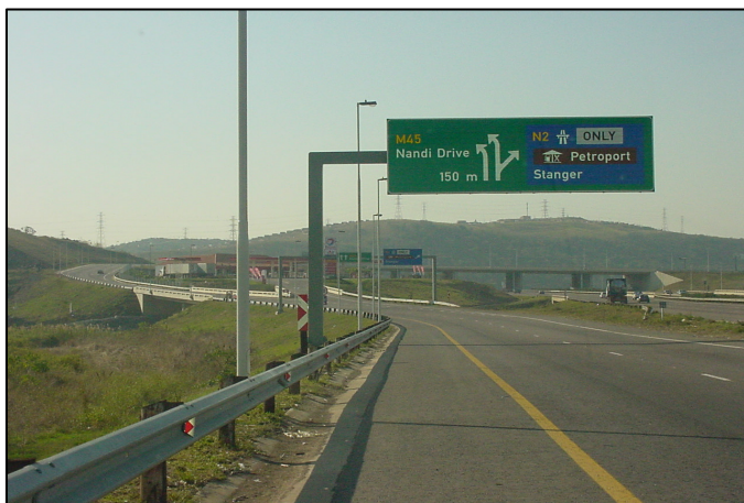
Plate 9.1: Road infrastructure for Riverhorse Valley completed by the eThekweni Municipality
