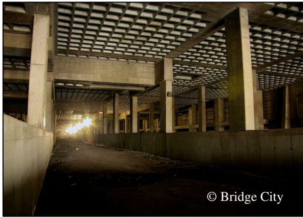
Plate 9.4: Construction of the new rail terminus at Bridge City
