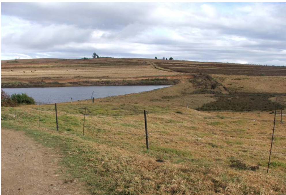
Figure 4.1 View of Killarney farm, 15 June 2006.
