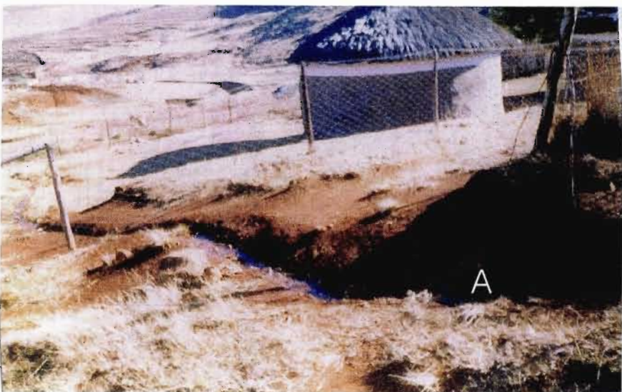
Fig. 5.4.2. A = heavily eroding furrow
