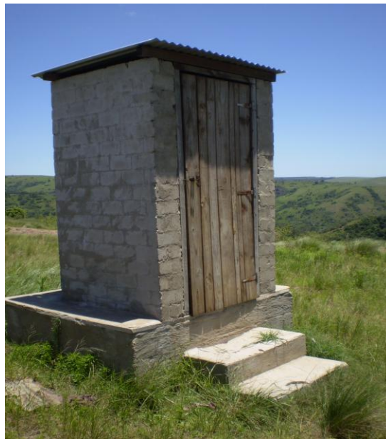
Figure 2.1: Operational urine diversion (UD) toilet in eThekweni Municipality, Durban (source: David Hawksworth).
