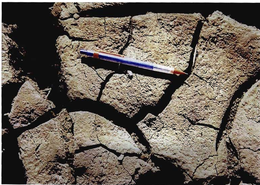
Figure 5.11 An example of polygonal cracking within the 'Stagstones' wetland. This constituted the most extreme cracking noted.
