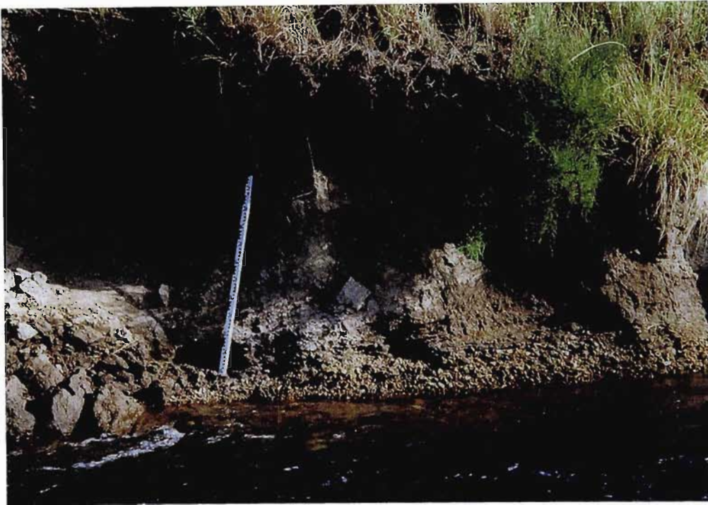
Figure 5.10 Section of channel bank recently collapsed as a result of high pore pressures, together with probable undercutting by flowing water.
