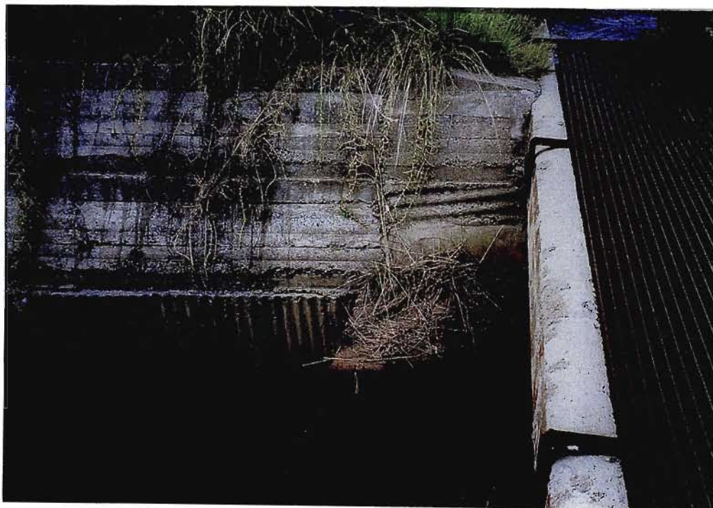
Figure 5.9 An example of a water way diversion (above the Mooi River), through which water is being channelled into trout dams.
