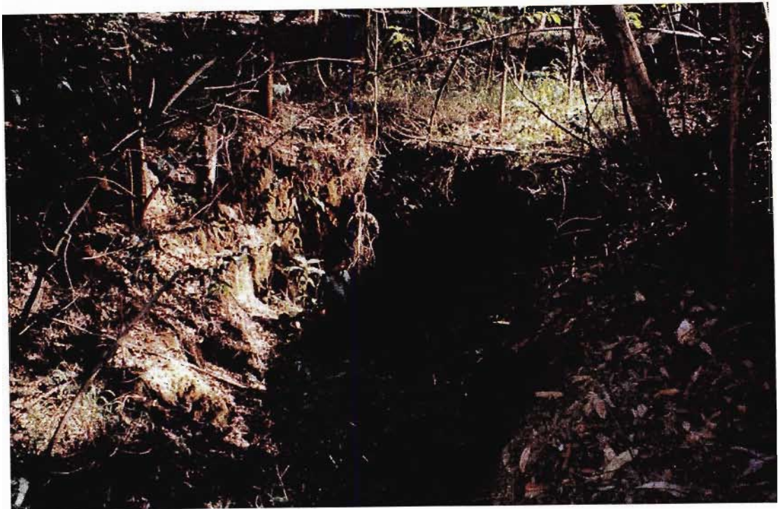
Figure 3.10: Onset of gully erosion at photo point 3
