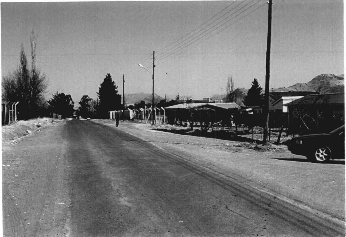
Plate 4.1 A section of Maseru West
