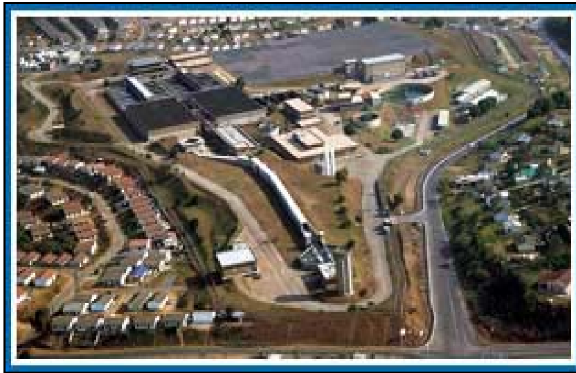
Figure 1-2: Wiggins Waterworks aerial view (Umgeni Water (2002))
