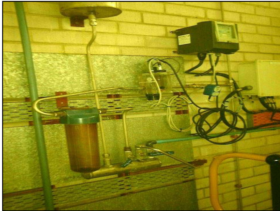
Figure 3-5: On-line pH meter, Chlorometer at the exit of the reservoir
