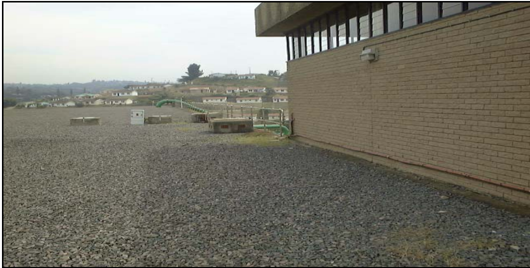
Figure 3-1: View of the top of the reservoir
