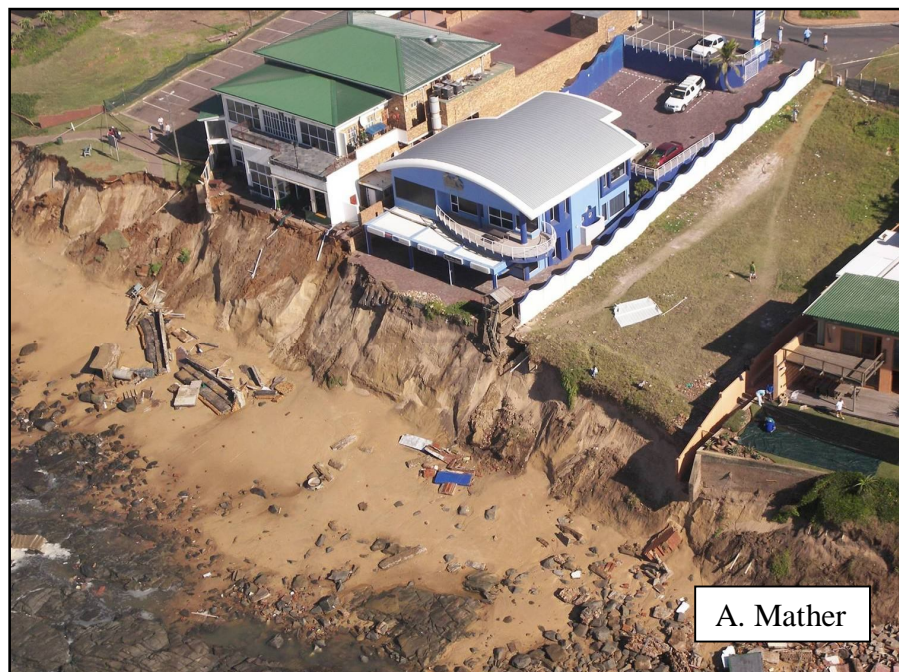
Plate 7: Destruction in Ballito (KZN) caused by the March 2007 storm surge event.
