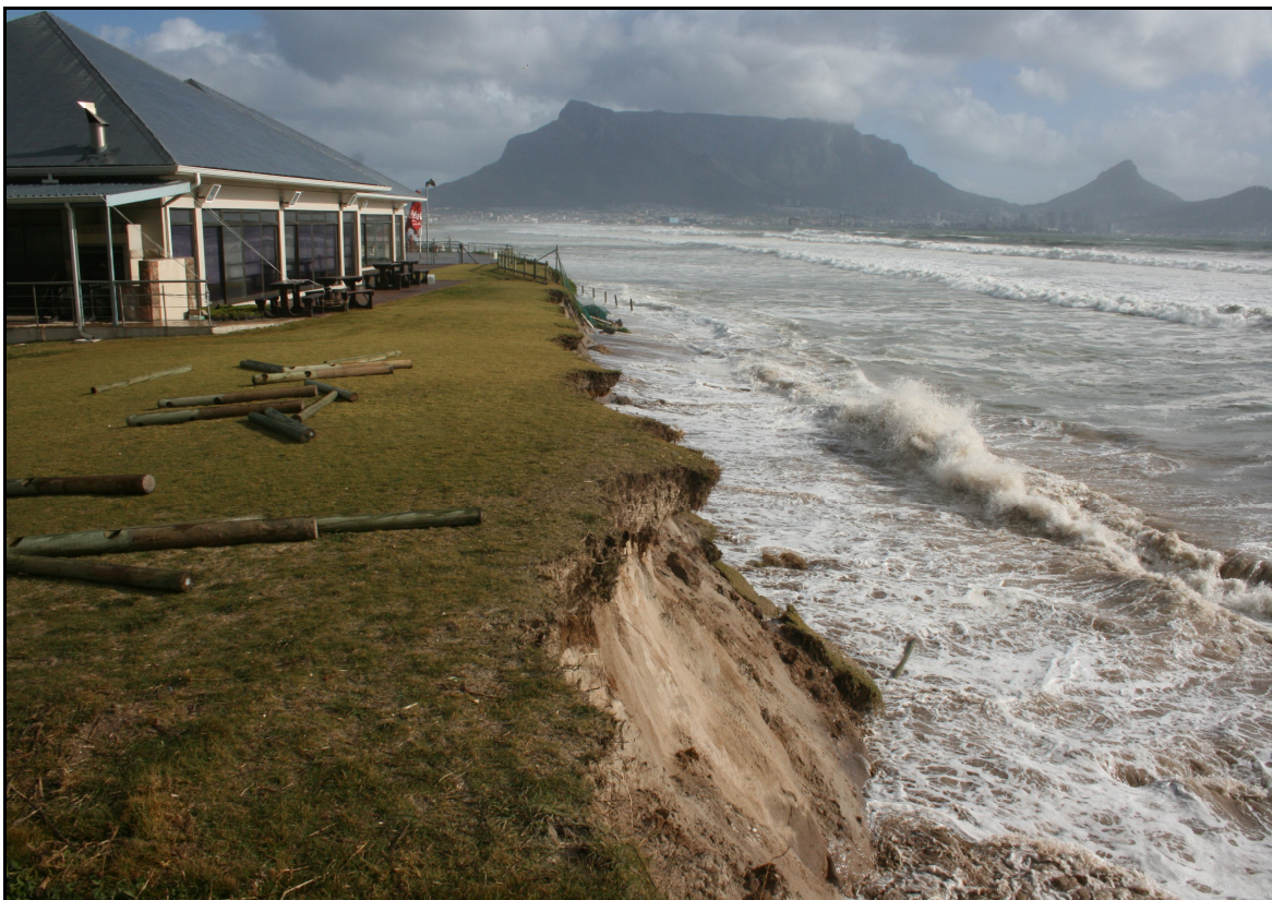
Plate 8: Milnerton Club House in Cape Town during the August storm surge event, 2008. Infrastructure at risk from storm surge events is a country-wide issue.
