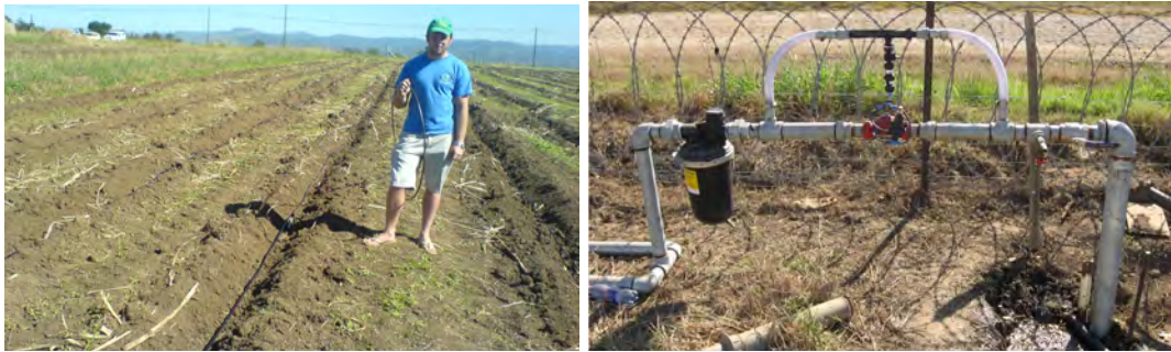
Figure 3.19 a) Drip tape installation
