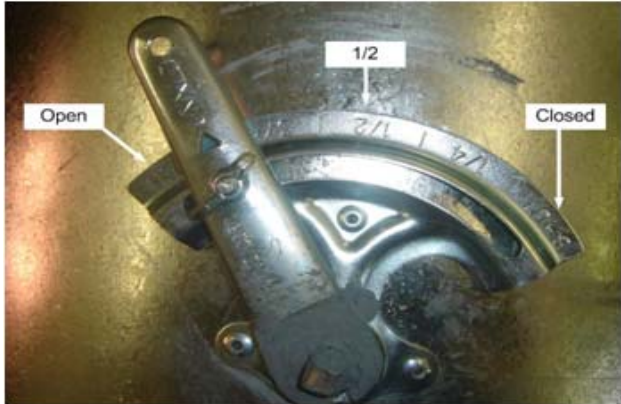
Fig. 7.3 Control mechanism of the inlet damper
