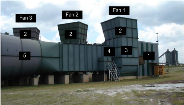
Fig. 1.2 Existing air ventilation system at Vlaklaagte
