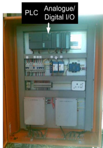
Fig. 10.3 PLC and interface equipment
