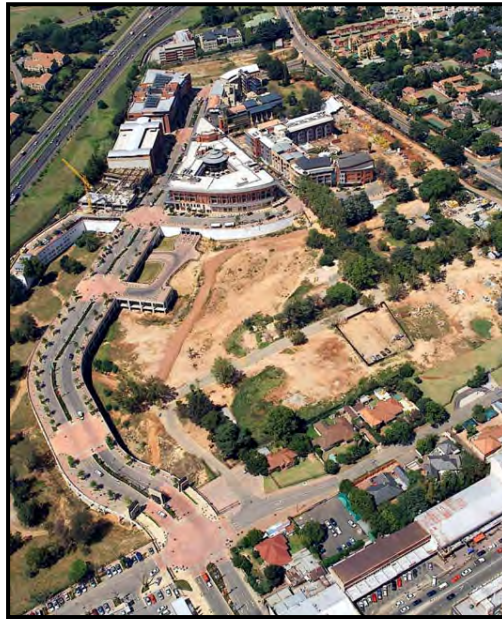
Figure 14 (above): Aerial image of the construction stage of Melrose Arch (www.arup.com)
