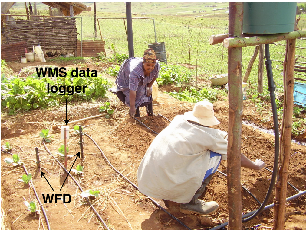
FIGURE 3.6: Site S2tb (right, 260 cm x 110 cm by 60 cm depth) and S1n (left, 260 cm x 130 cm), November 2006. Drip irrigation system installation over control bed and trench bed.
