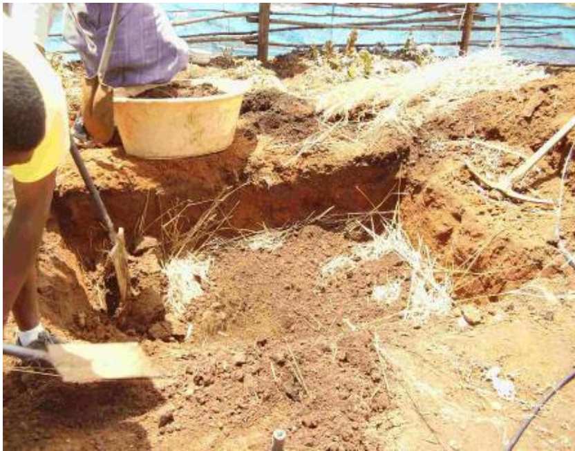
FIGURE 3.4: Placing trench bed fill.
