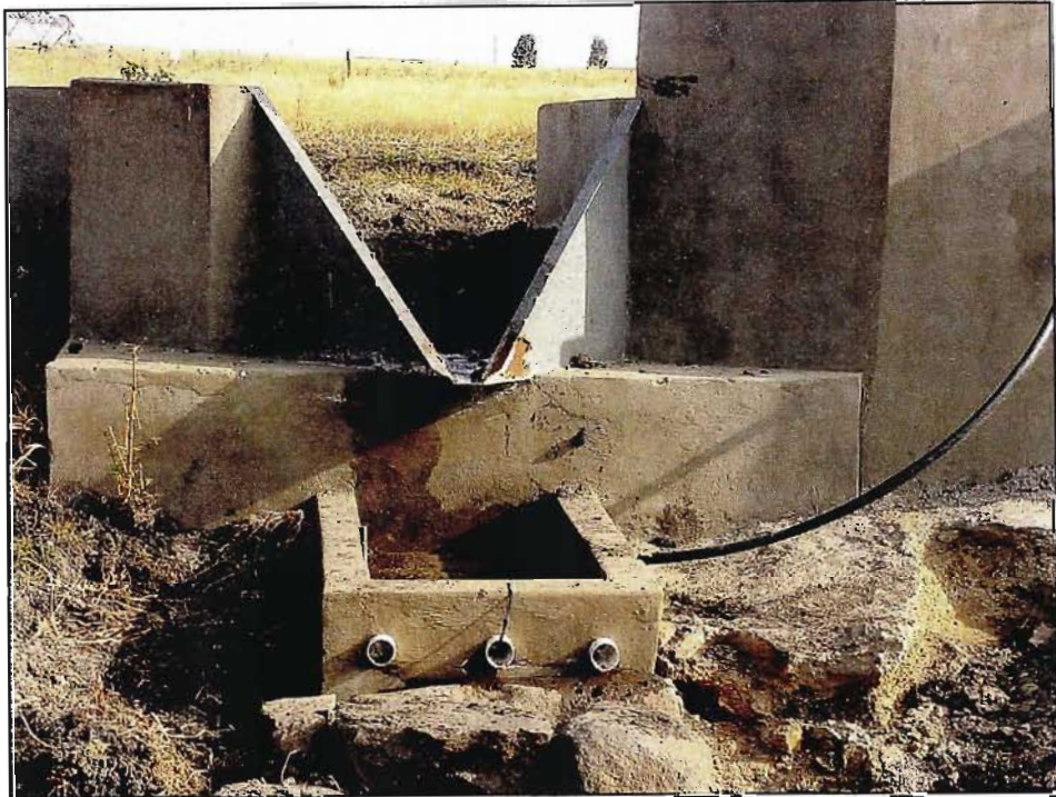
Figure 4.2: Syferfontein H flume
