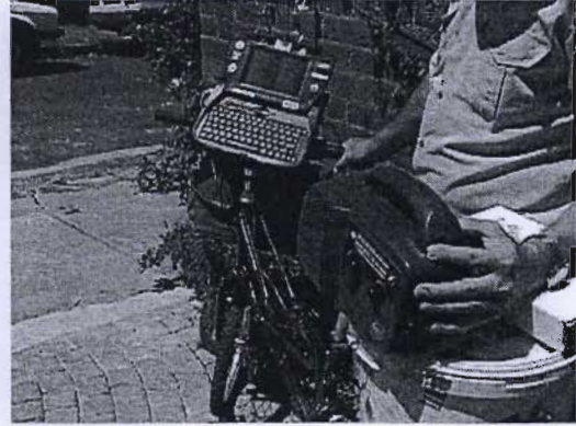
Folding mountain bike equipped with laptop, GPS, Cell Phone and Radio with integral power generator.
