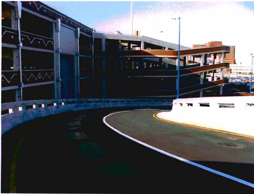
Plate 2.1: Overhead Double Carriageway Linking the Car Park at the Durban Car Terminal with the Quayside. (Photo courtesy of Terry Hudson).
