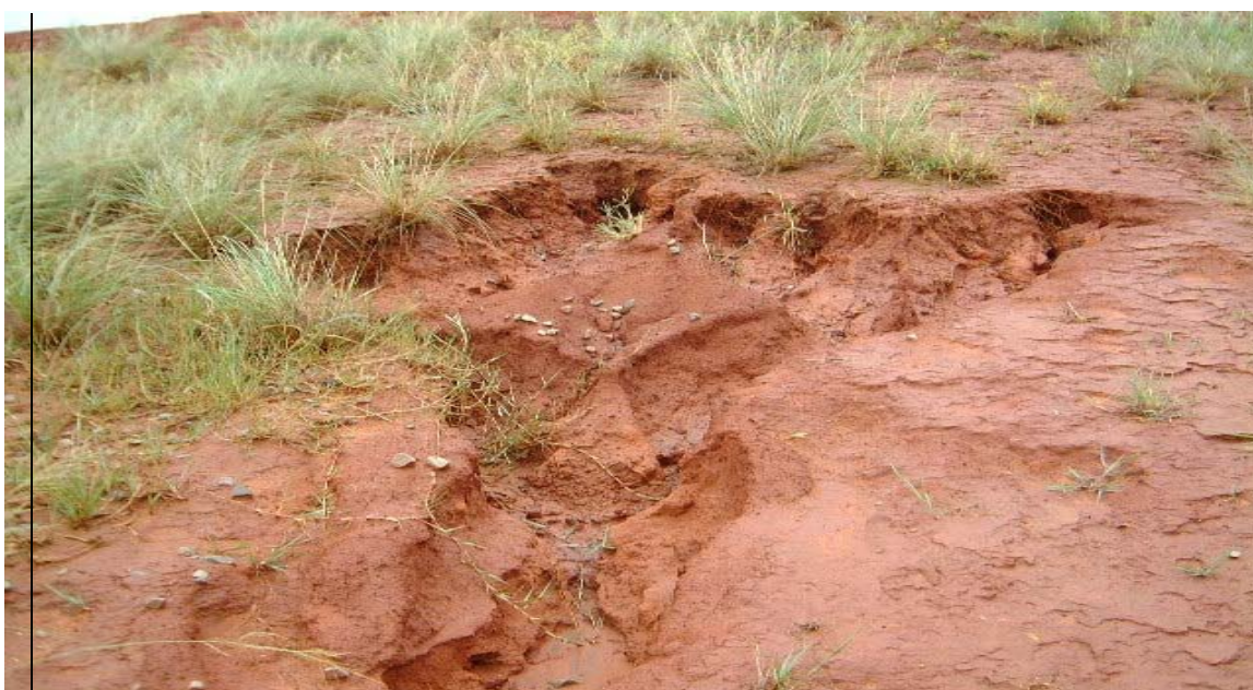
Figure 1.9 Excessive Erosion on previously capped area, affecting an estimated 40% of the south cell
