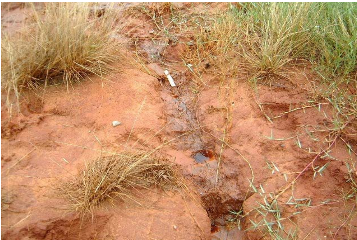
Figure 1.8 Formation of gullies and flow of leachate, affecting an estimated 25% of the south cell
