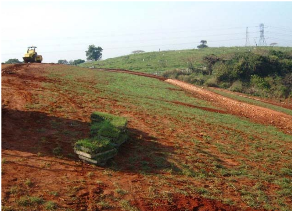
Figure 1.19 Cynodon dactylon plugs being planted and subsequently spreading on a landfill slope
