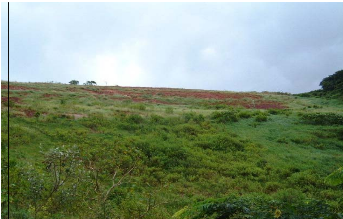
Figure 1.6 South side of landfill: methane eroded areas and lack of vegetation probably due to gas emissions
