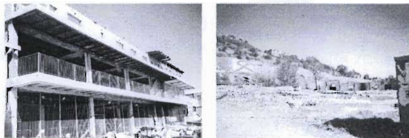
Figure 3: Retail Activity Site not yet Reconstructed
