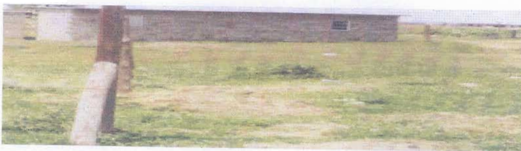
Plate 8 shows an informal house in the middle of an earth road. The poles indicate a line beyond which, on the right, no structure should have been erected
