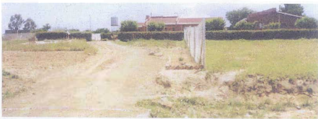
Plate 6 shows blocked access to a residential Lot. Here one has to go through another's property in order to gain access to his property
