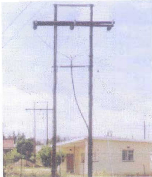
Plate 9 shows an informal house, which is imposing on electrical poles and cables
