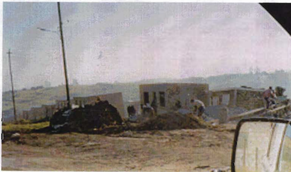
Fig. 4.4.3f Community engaged in blockmaking
