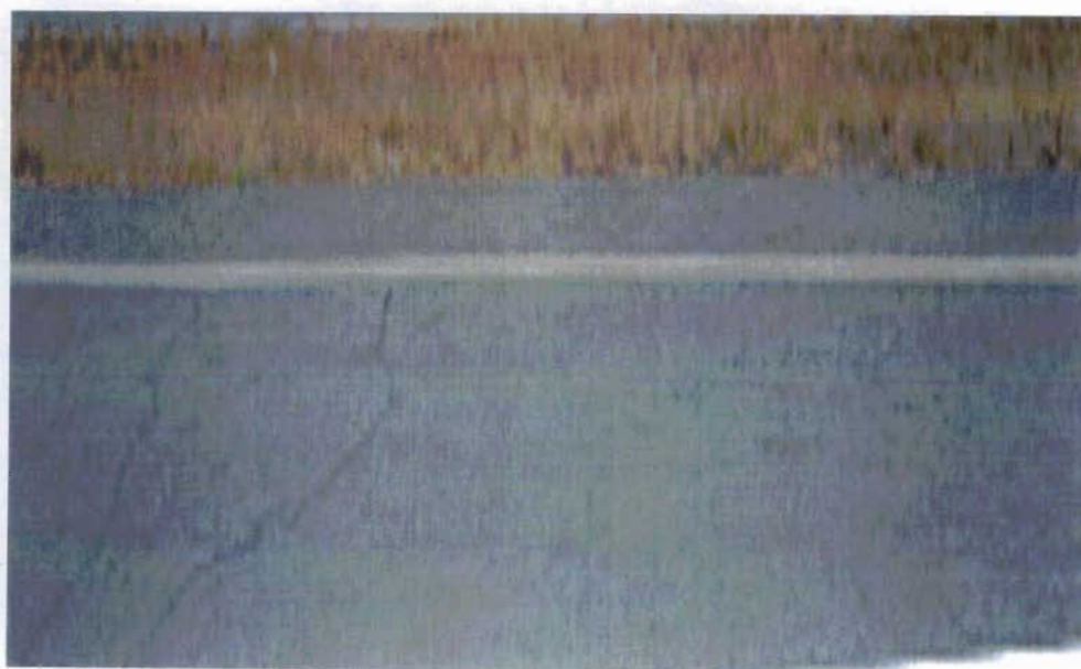
Fig. 4.5.2b Improved road in Dimbaza South after SPF intervention
