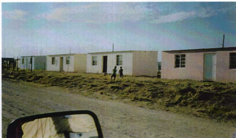
Fig. 4.5.2a Road in Dimbaza South prior to SPF intervention
