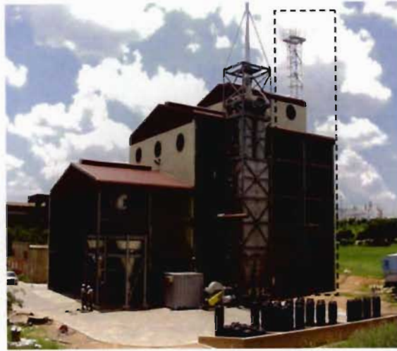
Figure 1-1 The Fluidised Bed Test Facility (FBTF), (Area enclosed by the dotted rectangle)
