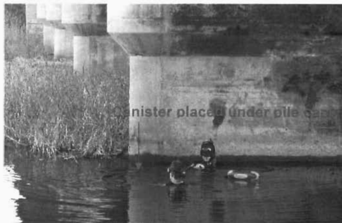
Plate 3.2 Water level logger deployed by divers under the pile cap of the northern, seaward side of the M4 bridge.
